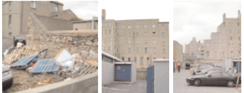
Back land and dereliction and underused urban land off Sussex Street
