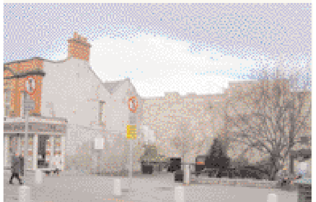
Gable end of EBS building
