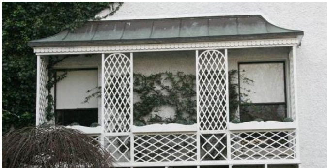
Oriel veranda at No. 8 Waltham Terrace
