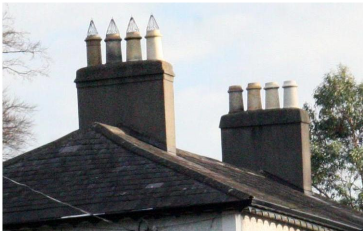
Typical chimney stacks and pots
