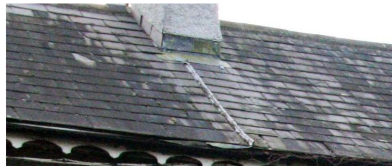
Detail of roof showing wider slates at eaves
