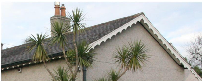
Typical decorative barge and eaves boards
