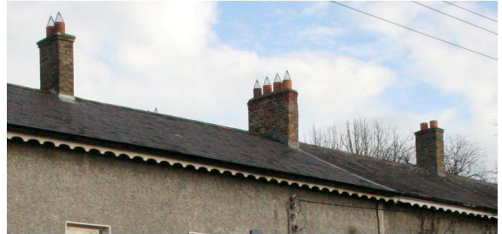
Brick chimney stacks
