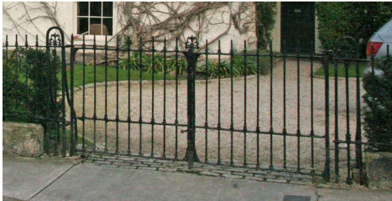
Iron gates and piers at No. 9 Waltham Terrace
