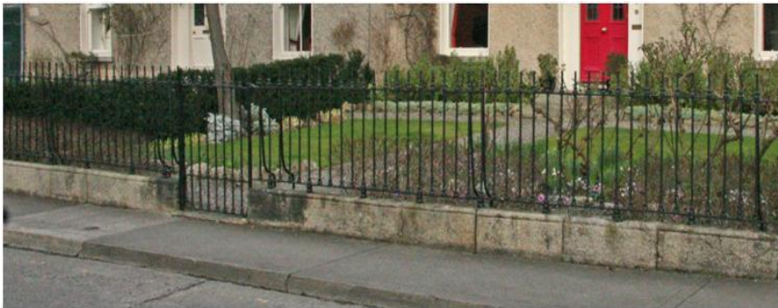
Typical plinth wall and railing
