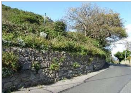
Stone retaining wall to Sorrento Park
