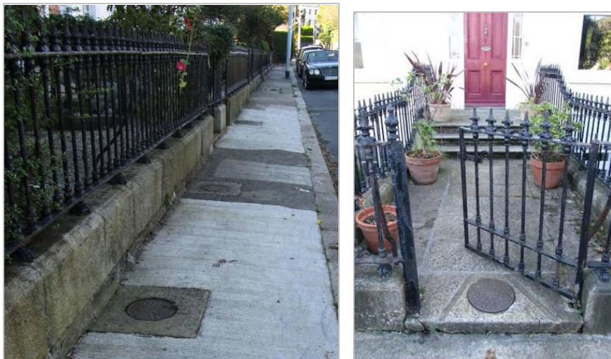
Left: coal covers in footpaths to basements in Sorrento Terrace Right: coal covers in stone garden paths in Sorrento Terrace
