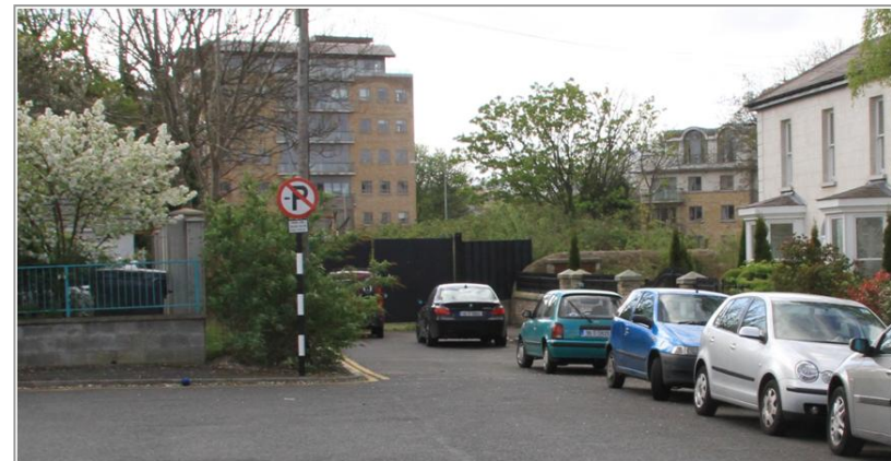
Plate 1: View towards vacant site at southern end of Sydenham Villas
