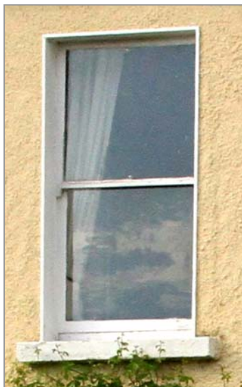
Plate 6: Detail of window, with rippling in glass, Huntersmoon.
