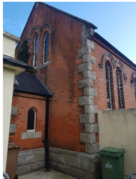
Photo 4: Entrance Porch & Western Gable
