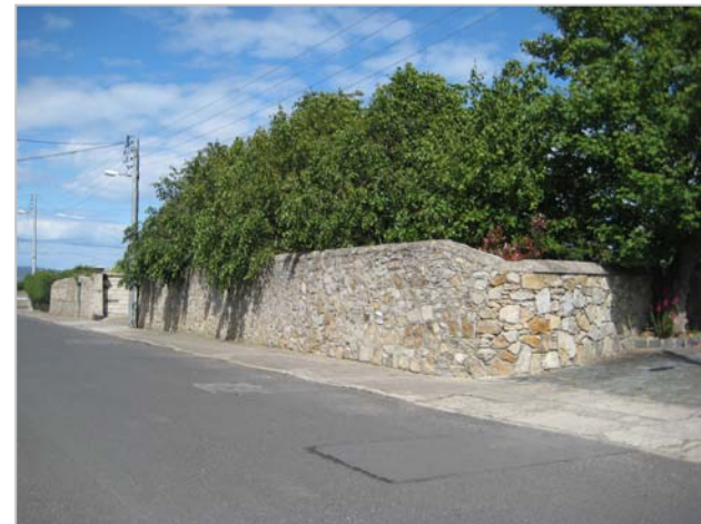
Granite rubble boundary wall
