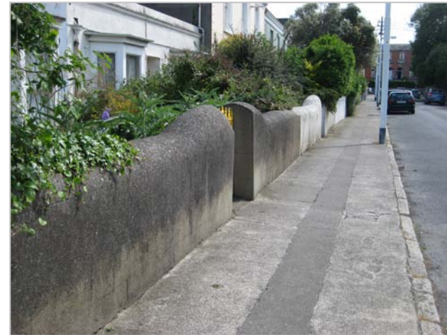
Cement-rendered boundary walls broken only by pedestrian gate
