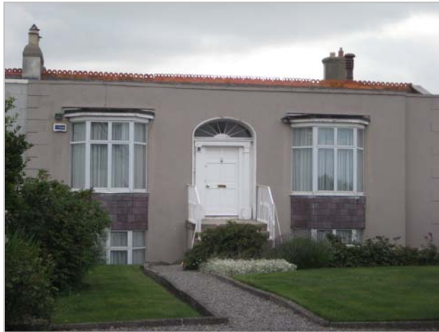
Inappropriate replacement windows.
