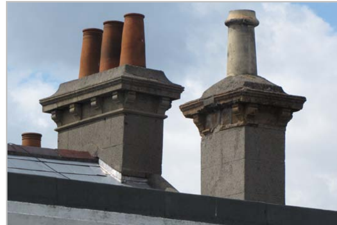
Typical cement-rendered chimneystacks
