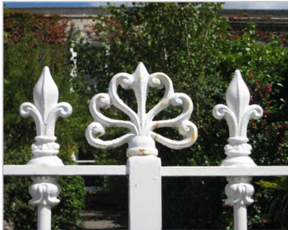
Cast-iron detail within the ACA
