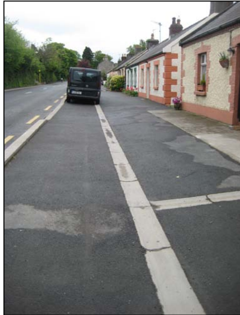
Photo 4: Tarmac surfacing to front of cottages
