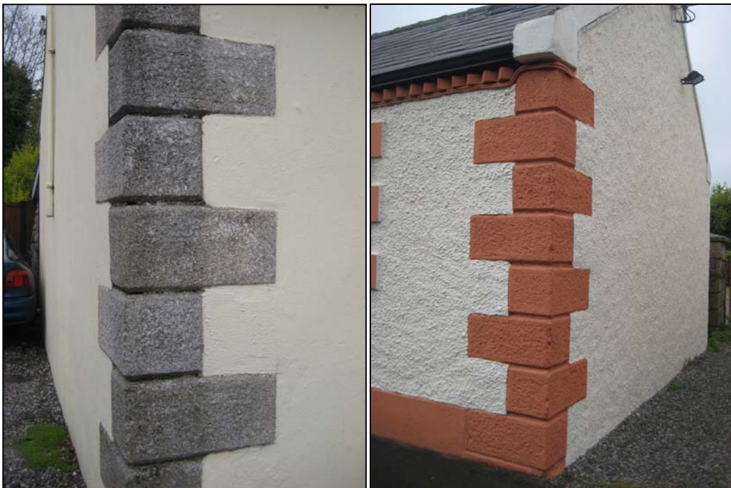
Photo 5 and 6: Exposed granite quoins in original state and later painted quoins
