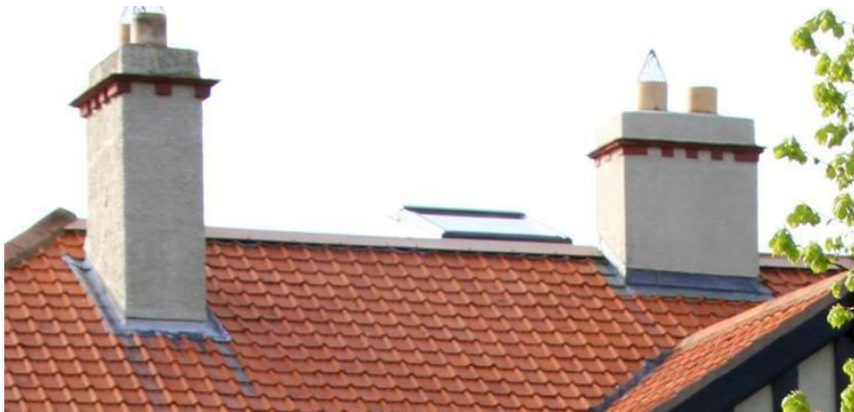
Typical original chimney stacks and plain pots
