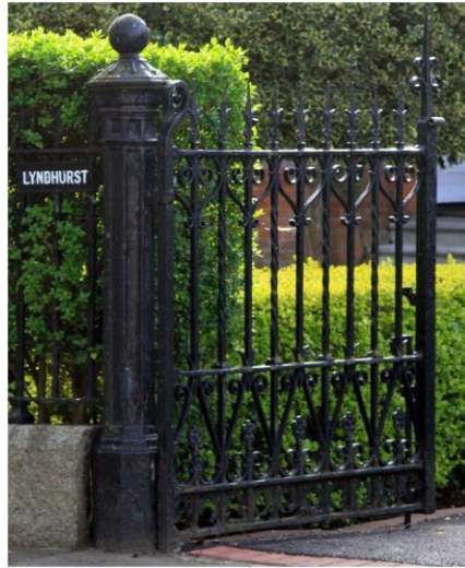
Railings, piers and gates at Lyndhurst
