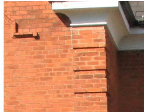
Detail of brick at Lyndhurst
