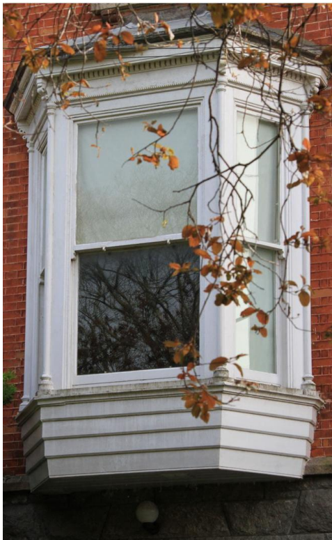
Oriel window at No. 1
