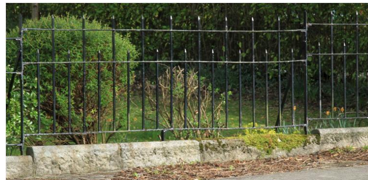
Typical wrought iron railings on rock-faced granite plinth
