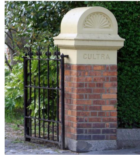
Pier and gate at Cultra
