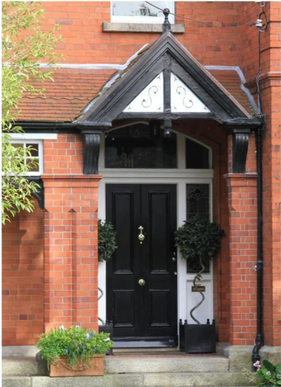
Porch at Hazelhurst
