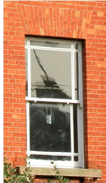
Window to side of No. 1 Marlborough Road
