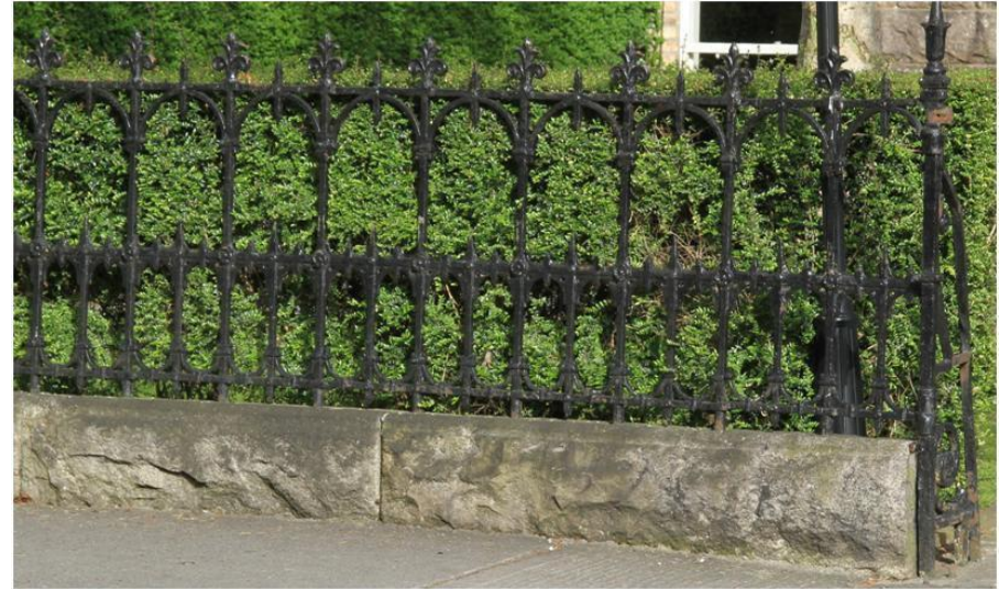
Cast iron railings at Lützen
