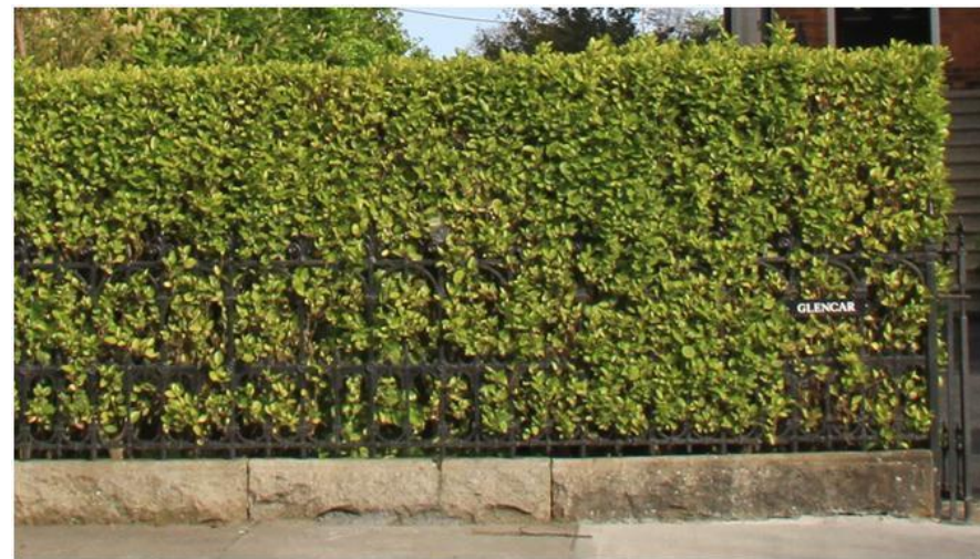
Iron railings on plinth wall, with hedge
