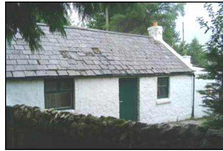
Vernacular Cottage, Barnacullia Historic Settlement Node
