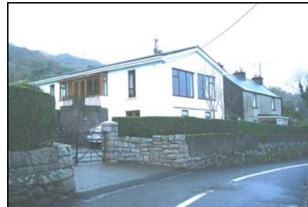
House, Barnacullia Historic Settlement Node
