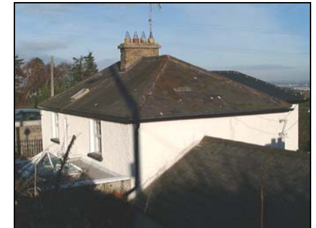
Double Storey Victorian House, with Hipped Roof, and Extensions, Ballyedmonduff/ Barnacullia Road Axis.
