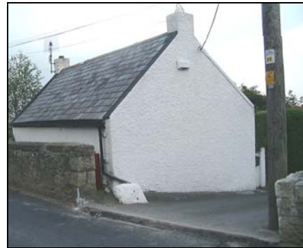
Vernacular Cottage, Barnacullia Historic Settlement Node
