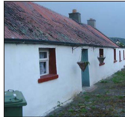
Vernacular Cottage with Metal Sheeted Roof, Barnacullia Historic Settlement Node
