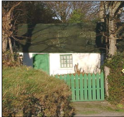
Vernacular Cottage with Metal Decked Roof, Ballyedmonduff/ Barnacullia Road Axis.
