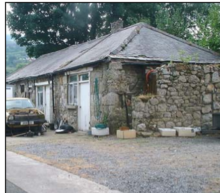
Stone Built Outhouses, Woodside House, Buffer Zone
