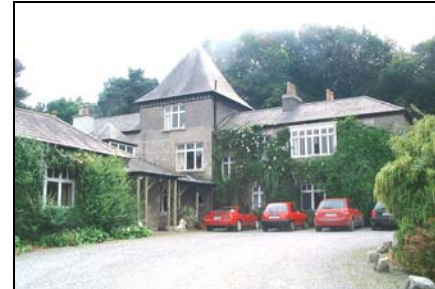
Fernhill House, Buffer Zone.
