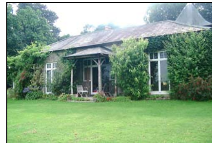
Fernhill House, Buffer Zone.
