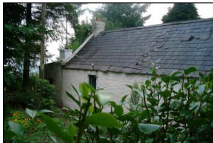
Vernacular Cottage, Barnacullia Historic Settlement Node
