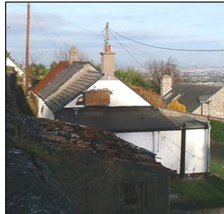
Vernacular Cottage, with additions, Ballyedmonduff/ Barnacullia Road Axis.
