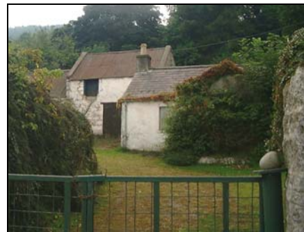
Vernacular Cottage and Double Storey Outbuildings, Barnacullia Historic Settlement Node
