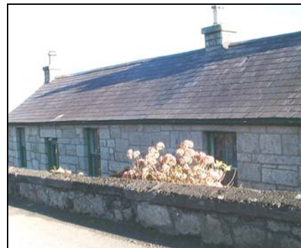
Vernacular Cottage with Cut Stone Masonry, Ballyedmonduff/ Barnacullia Road Axis.
