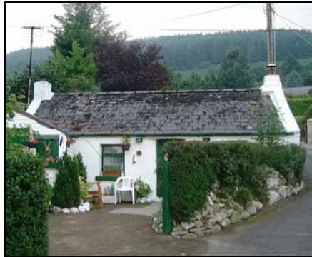
Vernacular Cottage, Barnacullia Historic Settlement Node
