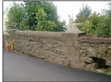
Bridge parapet, Ballyedmonduff / Barnacullia Road Axis
