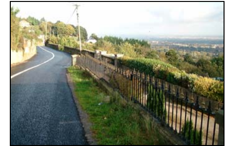
Metal Railings, Ballyedmonduff / Barnacullia Road Axis
