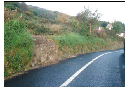
Stone Walling, Ballyedmonduff / Barnacullia Road Axis
