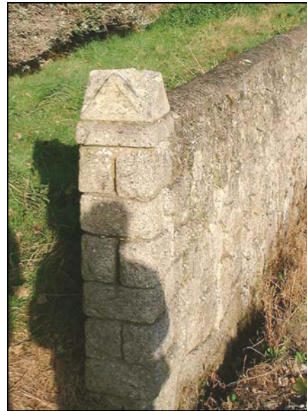
Gate Pier, Cul-de-Sac
