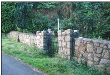
Gateway, Ballyedmonduff / Barnacullia Road Axis
