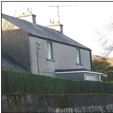
House Above Road Level, Ballyedmonduff / Barnacullia Road Axis
