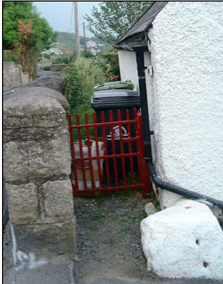
Gateway, Ballyedmonduff / Barnacullia Road Axis
