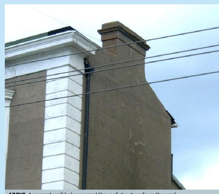
**ABOVE:** A parapet wall helps conceal the roof structure from the road
