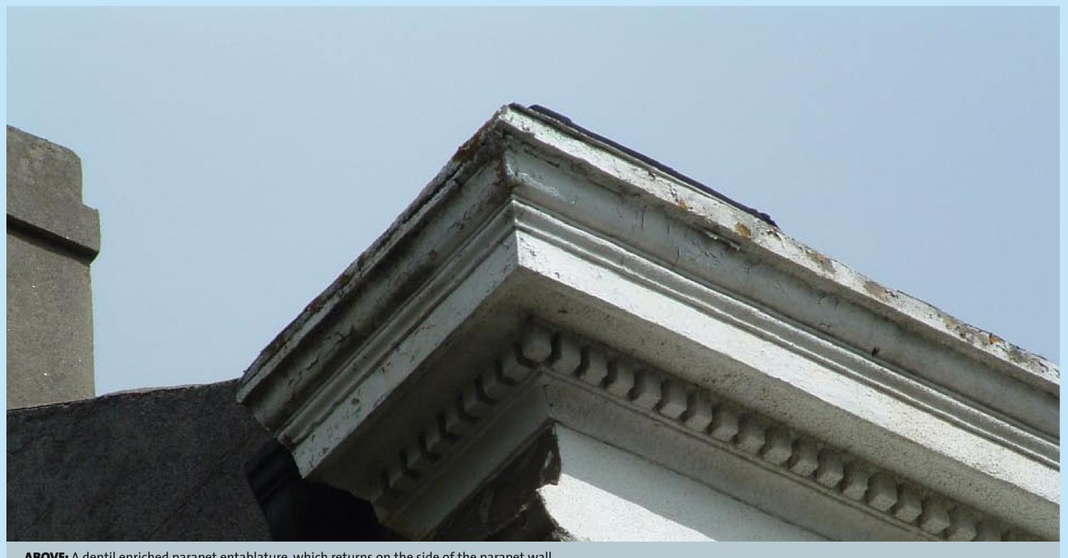
**ABOVE:** A dentil enriched parapet entablature, which returns on the side of the parapet wall
