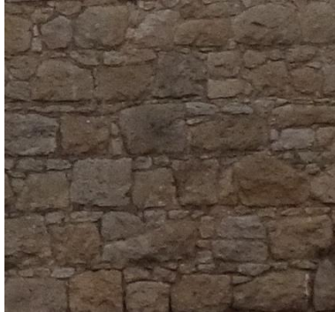
Photo 5.3: Granite rubble finish, Pembroke Cottages, Ballinteer Road
