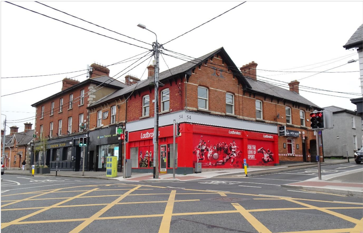
Photo 5.22: Dundrum House and Terrace
