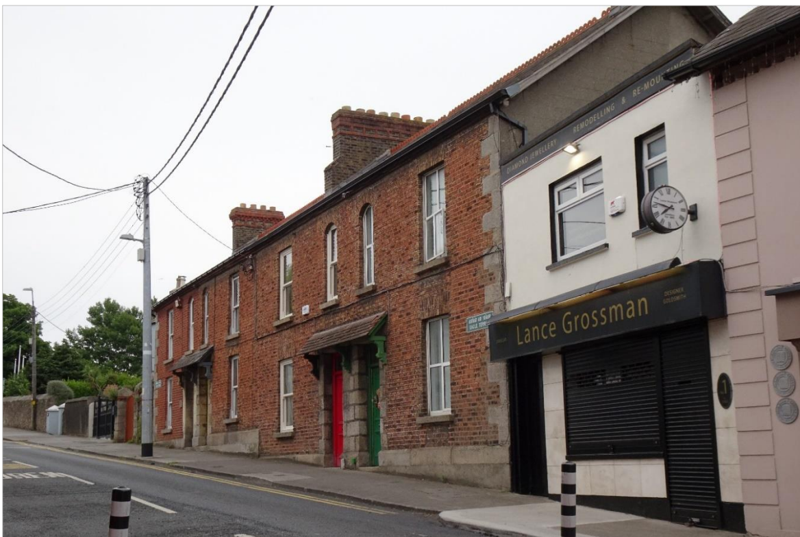
Photo 5.31: Eagle Terrace enclosing one side of the street on a steep incline along Kilmacud Road Upper.
