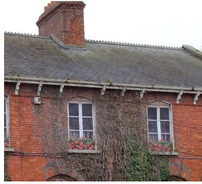
Photo 5.8: Use of slate at Glenville Terrace
