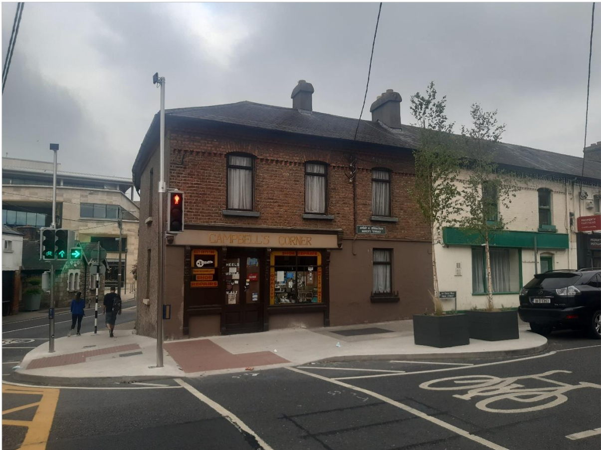
Photo 5.14 A view of a historic timber shopfront of the corner sited house forming the end of the Maher's Terrace.
