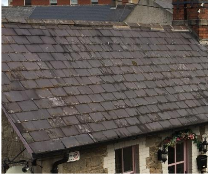
Photo 5.7: Slate in use at 1-2 Pembroke Cottages, Ballinteer Road
