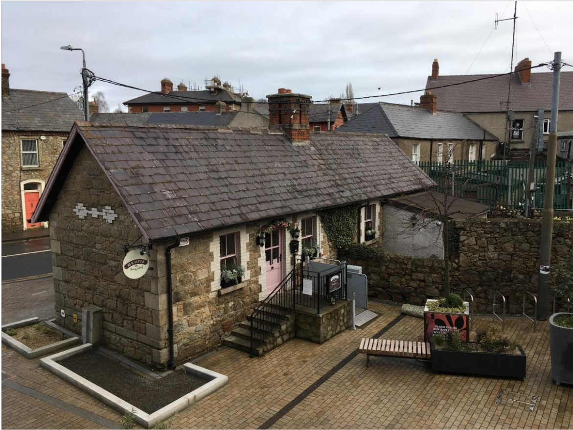
Photo 5.29: Rear view of Nos 1-2 Pembroke Cottages. The cottages front onto the Ballinteer Road.
