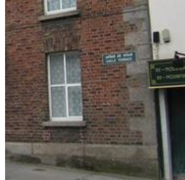
Photo 5.4: Granite dressing on red brick building, Eagle Terrace
