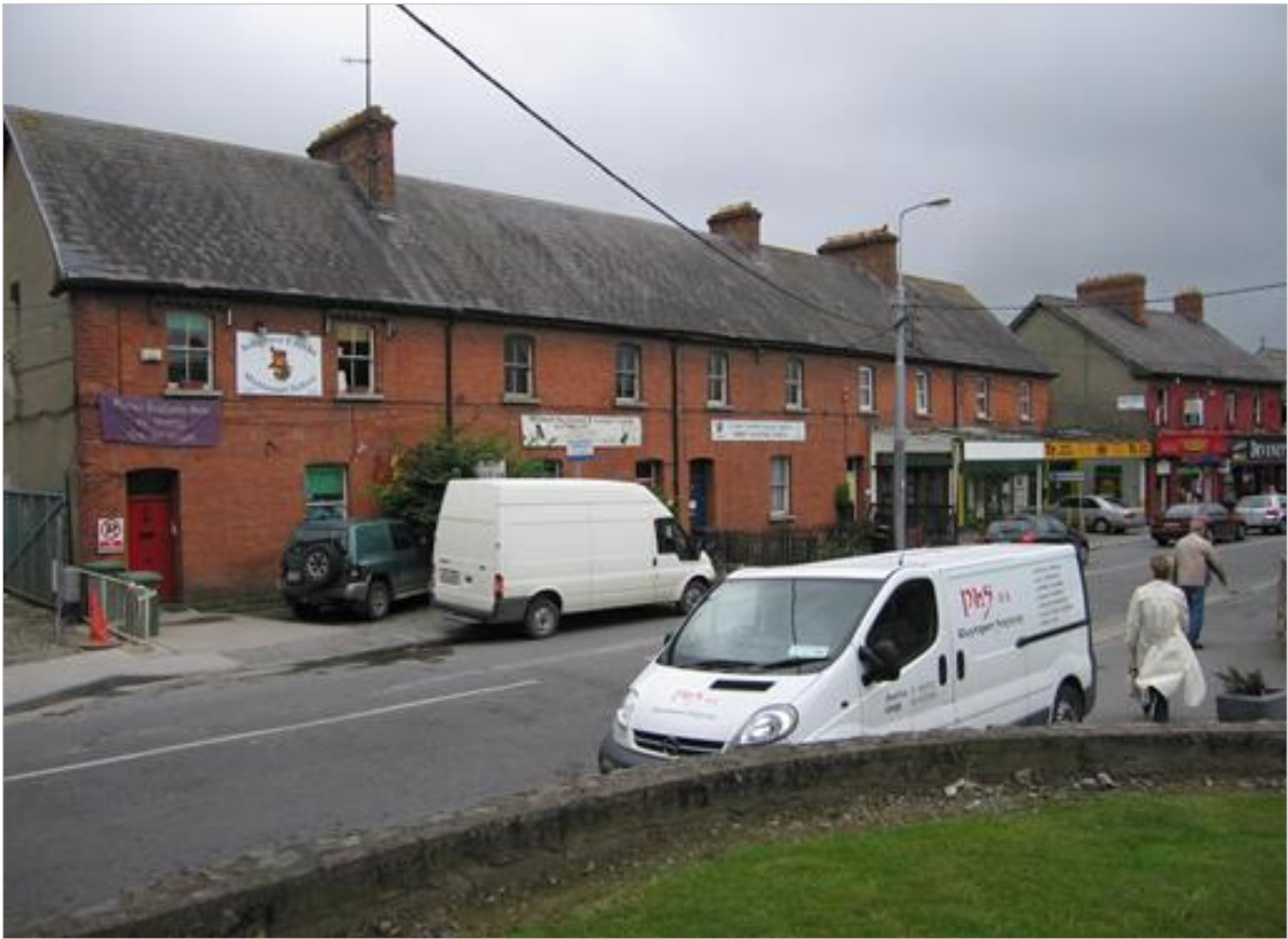
Photo 5.16: Ashgrove Terrace prior to refurbishment
