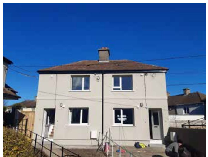
Eden Villas Refurbishment completed
