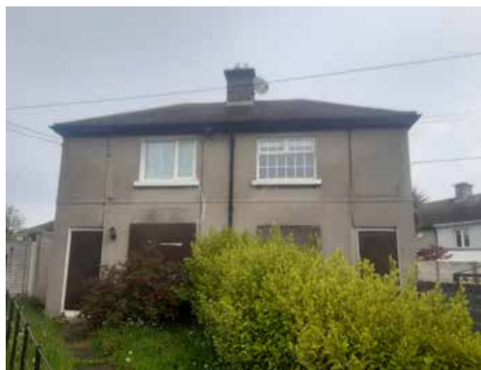
Eden Villas Refurbishment (before)
