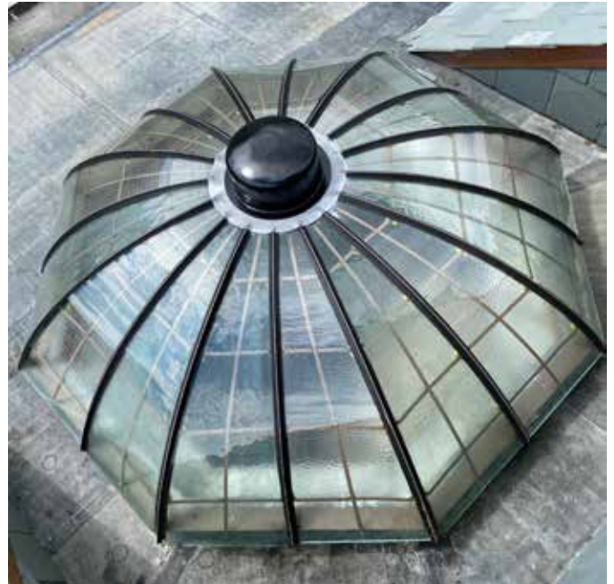
DL Carnegie Library Rooflight Repair (After)
