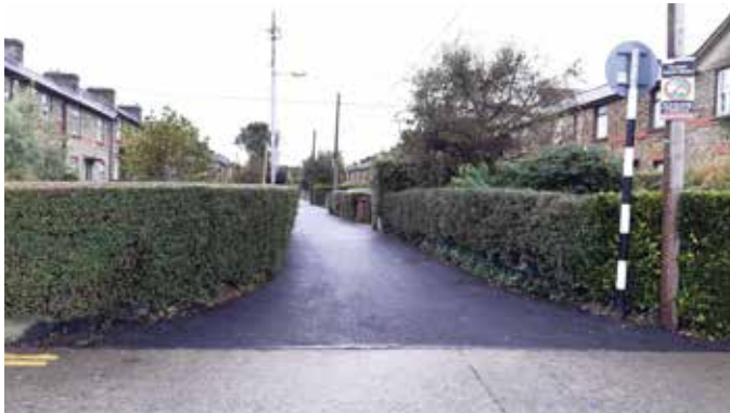
Roads Control - Reinstatement Works Devitt Villas
