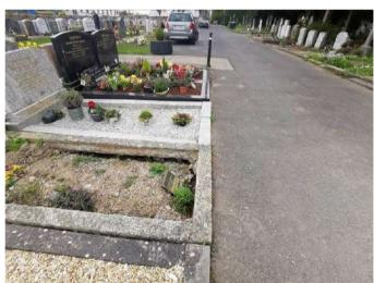
Plate 15 Subsidence and voids to burial plot adjacent proposed cycle lane route, facing south
