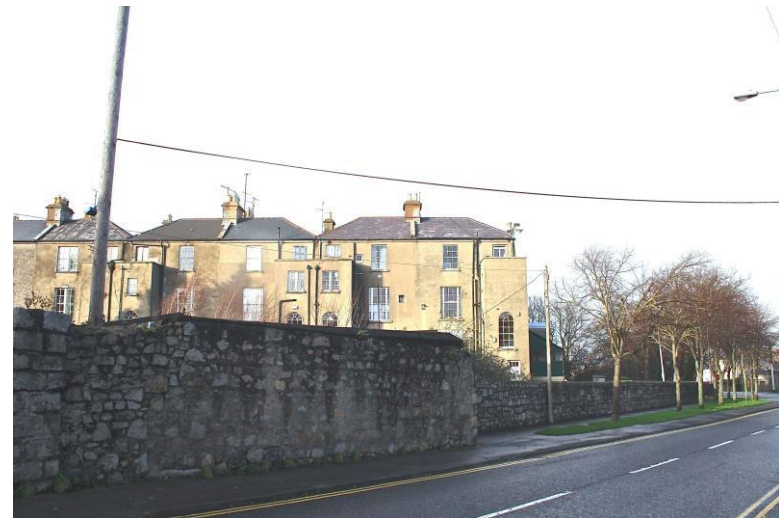
Rear roofscape Vesey Place
