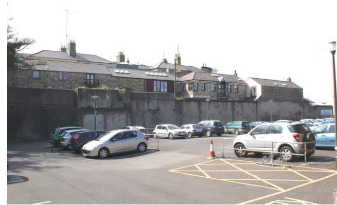
Retaining wall to rear De Vesce Terrace- view from VEC lands
