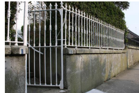
Railings and plinth wall De Vesce Terrace
