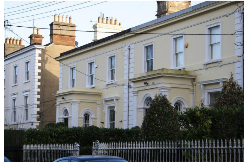
Wired services Vesey Place
