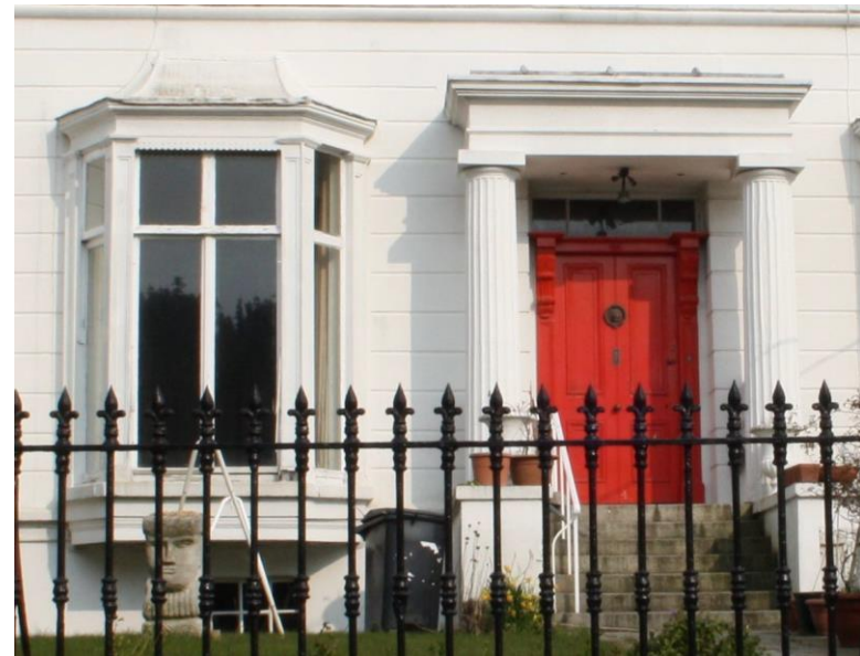
Oriel window and doorway De Vesce Terrace
