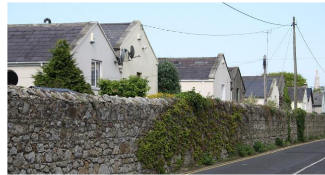
Wall to Vesey Mews- view from Knapton Lawn
