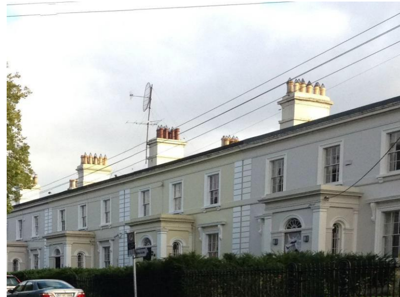
Chimney Stacks and Pots Vesey Place
