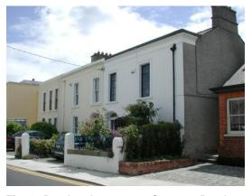
Fig. 18 Rendered terrace on Sorrento Road having moulded architraves and moulded Cornice to the parapet.
