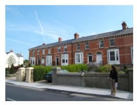
Fig. 17 Mid 19<sup>th</sup> century terrace on Ulverton Road using polychromatic brick, timber bracketed eaves and canted bays.
