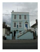
The mid 19<sup>th</sup> century building housing the Garda Station is a two-storey over raised basement structure with rendered elevation, moulded cornice to parapet and moulded entablature above the ground floor windows. A flight of granite steps returning with a quarter landing and flanked by wrought iron railings with cast iron finials leads to the front door with a carriage arch accessing the rear site.
