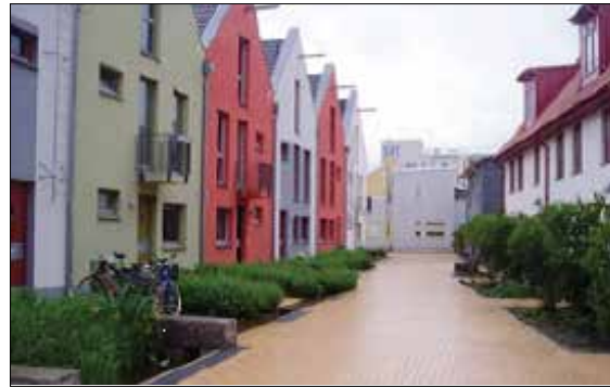
Figure 19 - Home-zone street in Malmo incorporating SuDS
