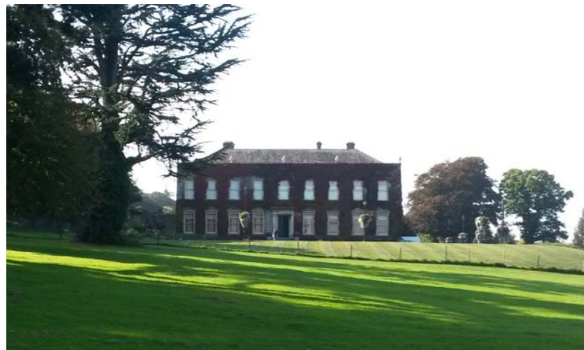
Photo 32: Cabinteely House, Cabinteely Park.
