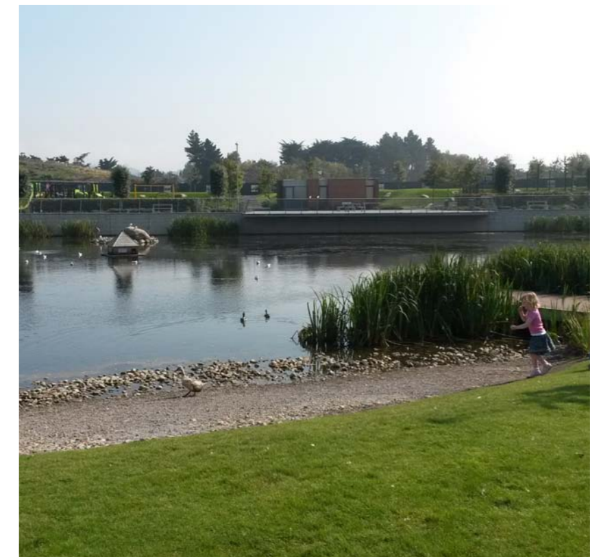
Photo 37: Attenuation Feature at Honeypark, Glenageary.
