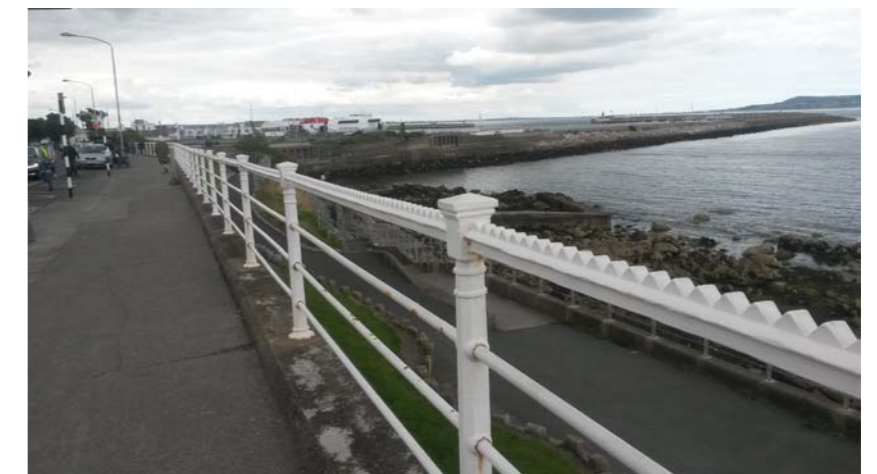
Photo 25: Railings along Queen's Road, Dún Laoghaire.
