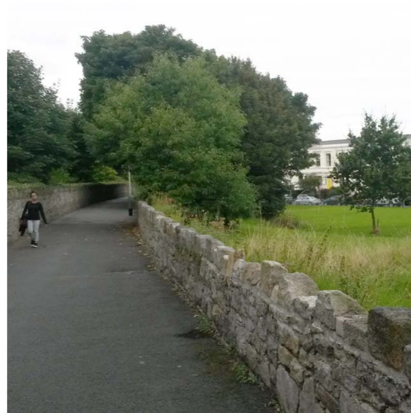
Photo 36: The Metals at Claremont Villas.
