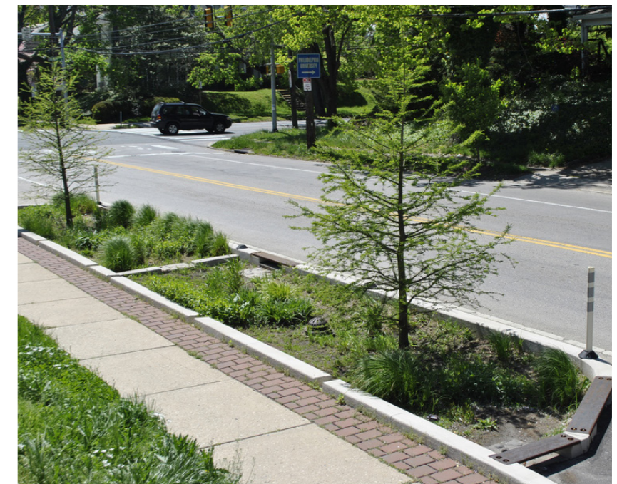
Photo 60: Stormwater Bump-Out on Queen Lane, Philadelphia. Source: Flickr. Image By: Philadelphia Water Department.
