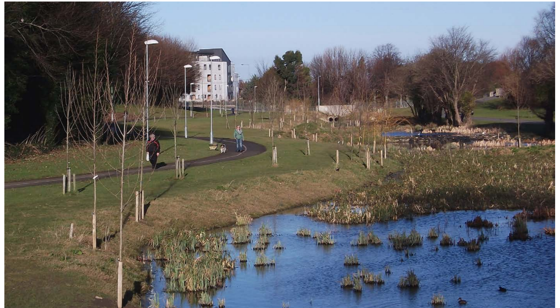
Photo 56: Kilbogget Park, Constructed Attenuation Wetlands Habitat.
