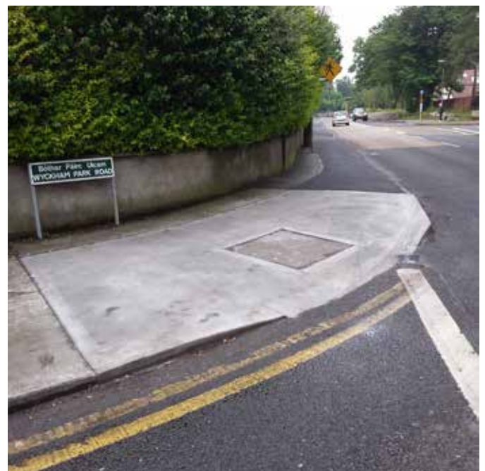
Road Maintenance Accessibility Improvement Works, Ballinteer
