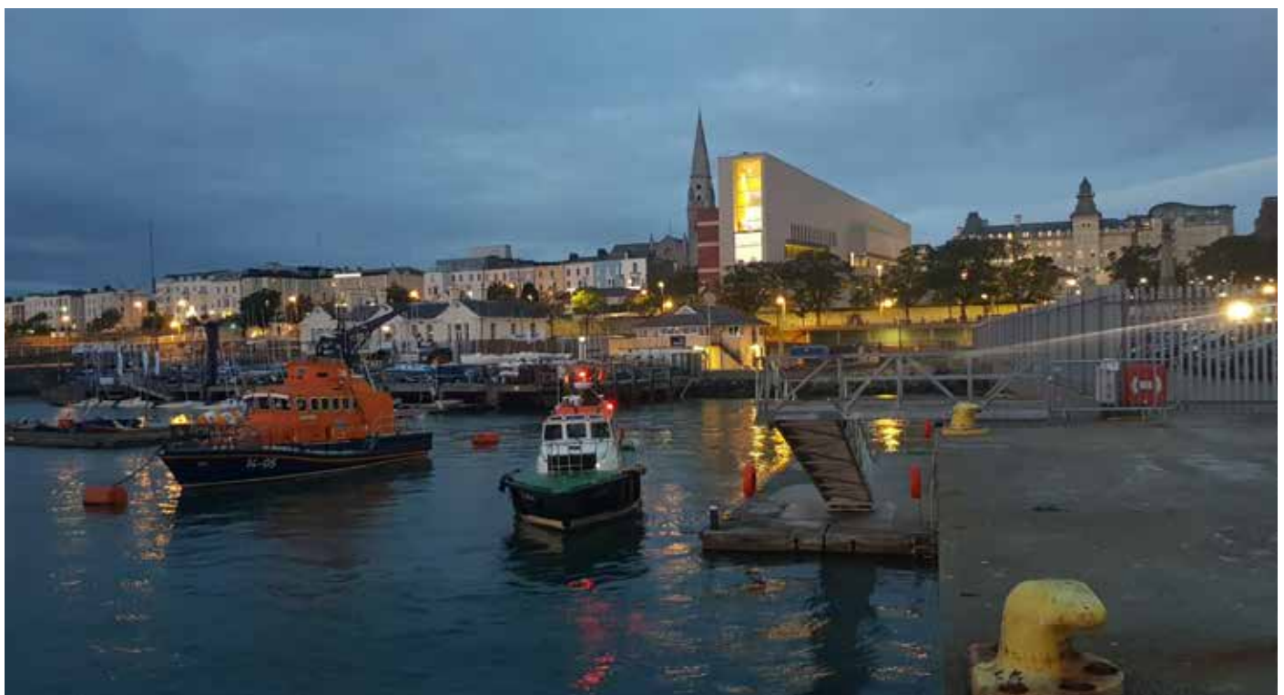
New Tender Berth Carlisle Pier, Dún Laoghaire
