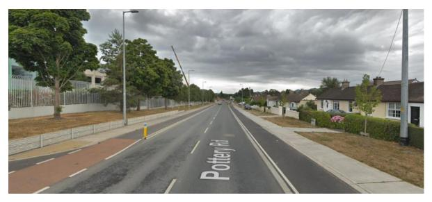
Figure 7-1 Example one-way kerb protected cycle track
