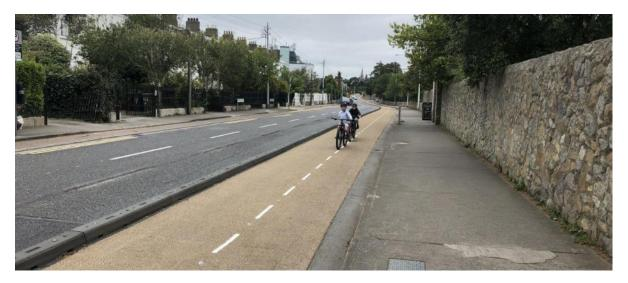
Figure 7-2 Example two-way kerb protected cycle track
