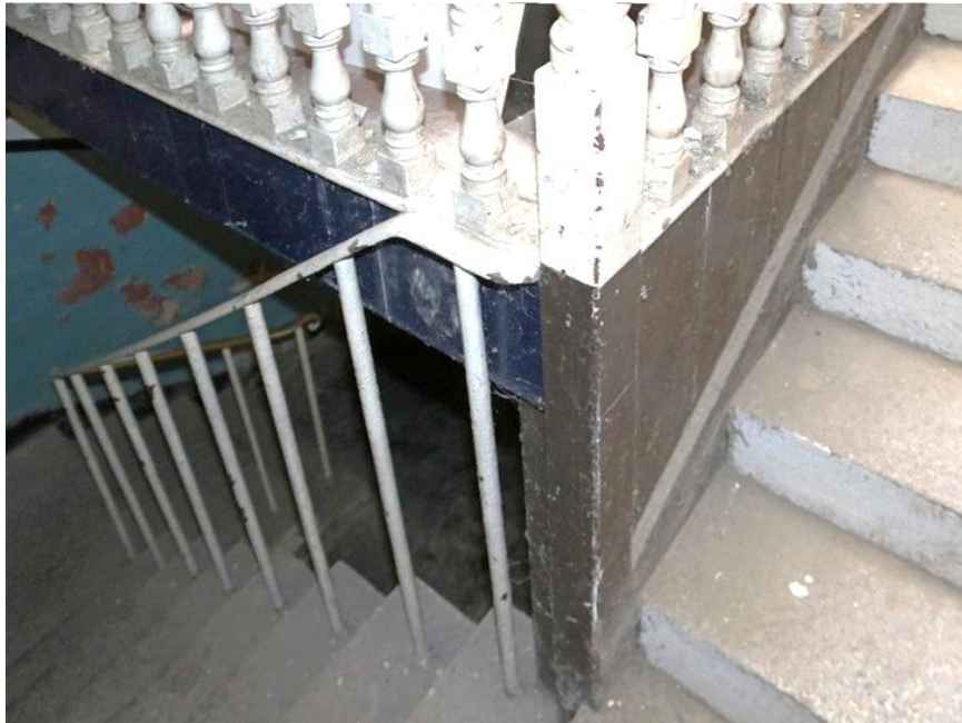
Plate 80: Iron balustrade on steps to basement
