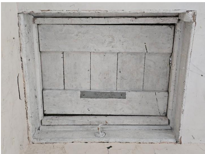
Plate 151: Trapdoor access in ceiling
