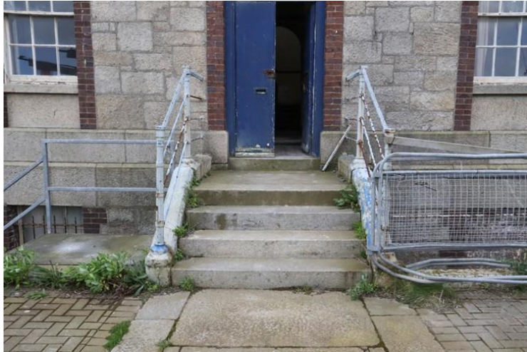
Plate 22: Granite steps leading to front door
