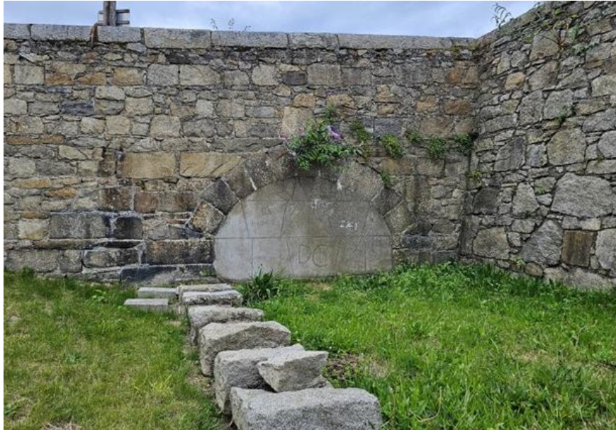
Plate 263: Arch of bridge beneath access ramp
