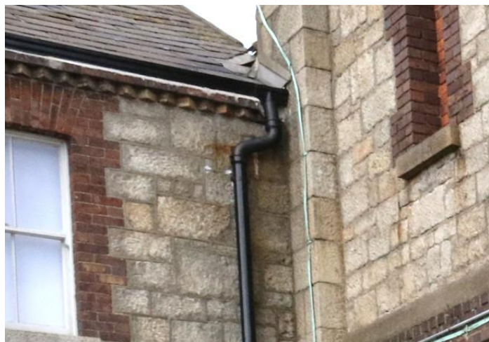
Plate 189: Swans neck and downpipe at house 8
