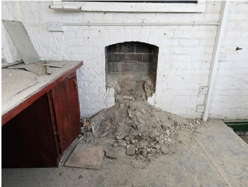
Plate 165: Hearth on second floor of tower
