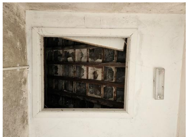
Plate 103: Trapdoor access to roof space
