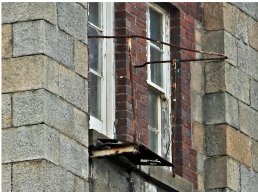
Plate 136: Balconette at northern window on second floor
