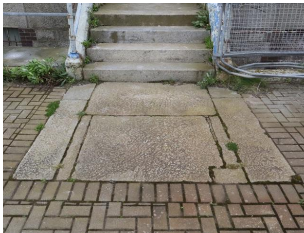
Plate 23: Granite flags at front door
