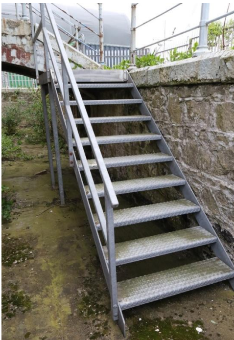
Plate 29 (left): Steel steps to basement area
