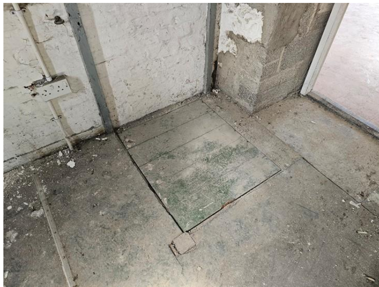
Plate 160: Trapdoor in floor at first-floor level
