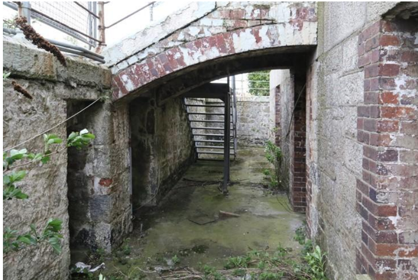
Plate 25: Arch carrying steps to front door of officer's house
