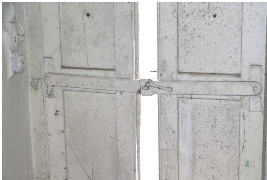
Plate 46: Wrought-iron fastenings at rear of shutters
