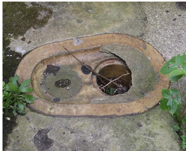
Plate 37: Drain and rodding eye
