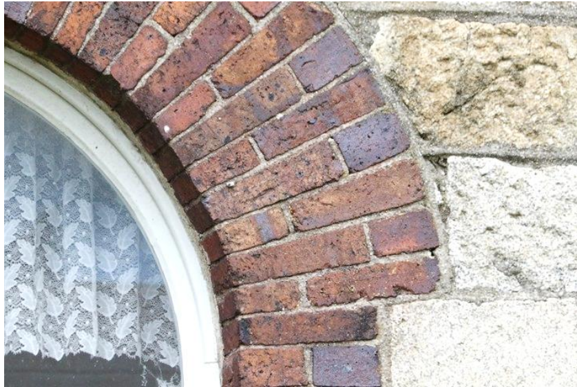
Plate 188: Detail of brick arch at window heads
