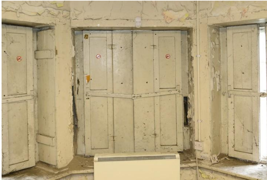
Plate 45: Shuttered windows in canted bay
