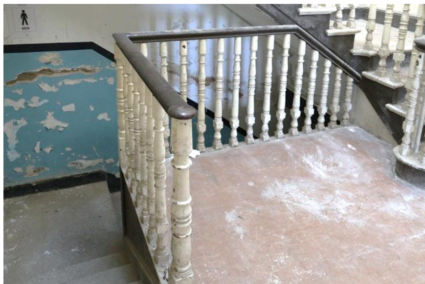
Plate 81: Timber balustrade at stairwell of basement stairs
