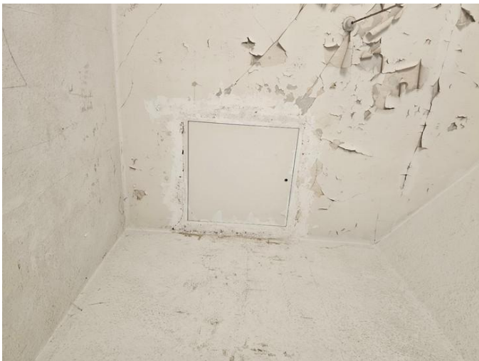
Plate 224: Access trapdoor in ceiling
