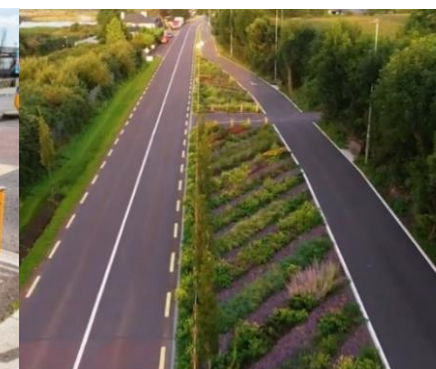
Figure 15-8 The Dunkettle to Carrigtwohill Cycleway Scheme, with SuDS in the form of a pollinator corridor. Source: Cork County Council
