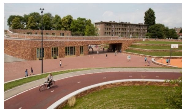
Figure 4-5 Integration of the approach span of the cycle route with the roof of the nearby primary school. Source: ARUP / Jeroen Musch
