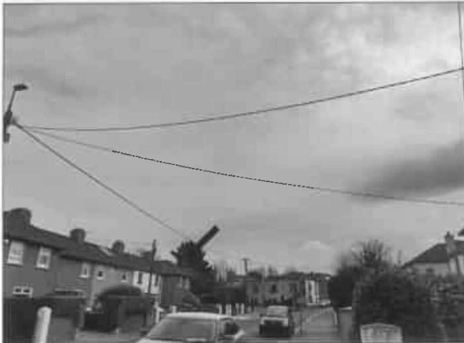
VRP9 - WITH SOLUTION IN PLACE
