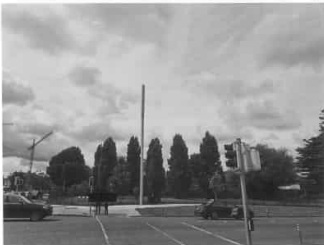
Fig 1. Existing Smart Streetpole Solution as erected in Drummartin Road, Kilmacud, Dublin 14.
