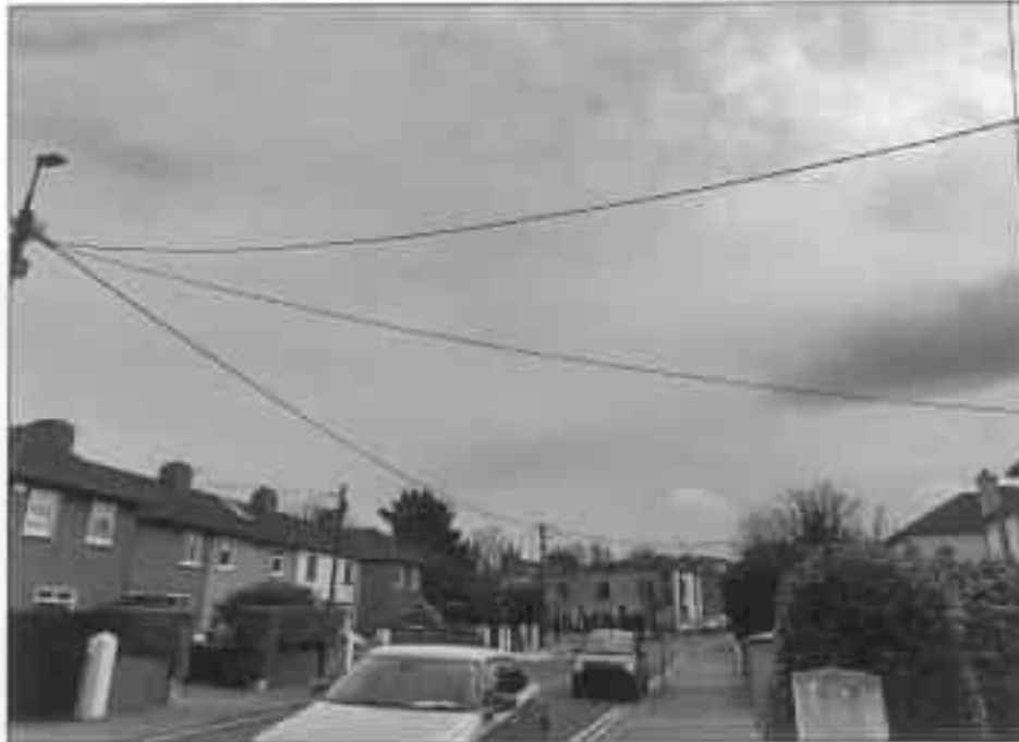
VRP9 - WITHOUT SOLUTION IN PLACE
