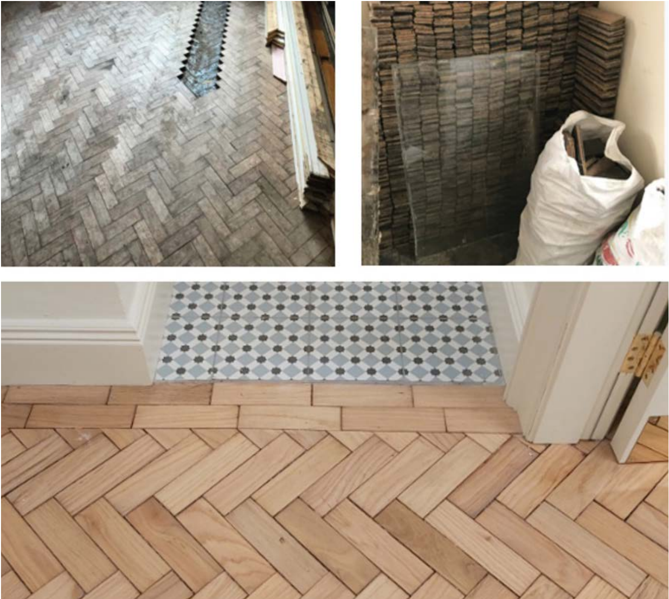
Figure 4-2: Reuse of flooring
