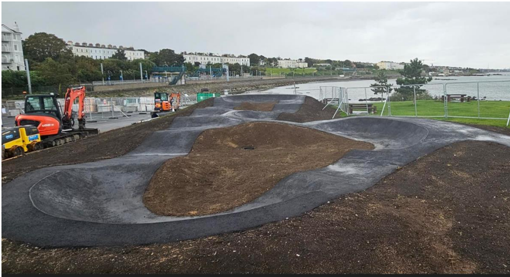
The Pump Track under construction in Apna Park
