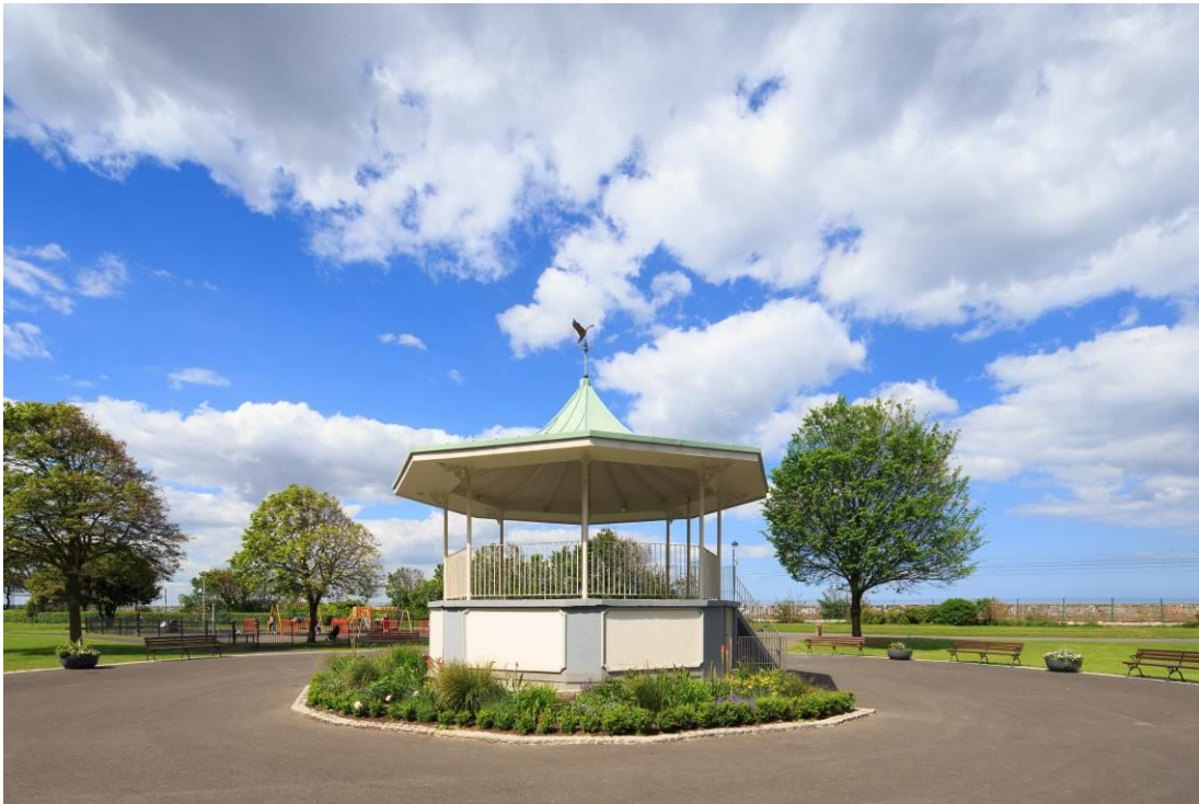
The restored bandstand surrounded by perennial planting which encourages pollinators and provides colour from late spring to early autumn.
