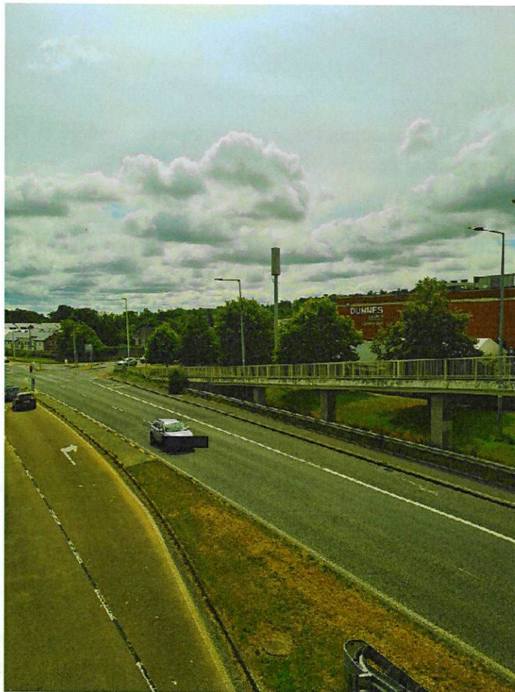
Fig 1. Existing Smart Streetpole Solution as erected along the N11, Cabinteely, Co. Dublin
