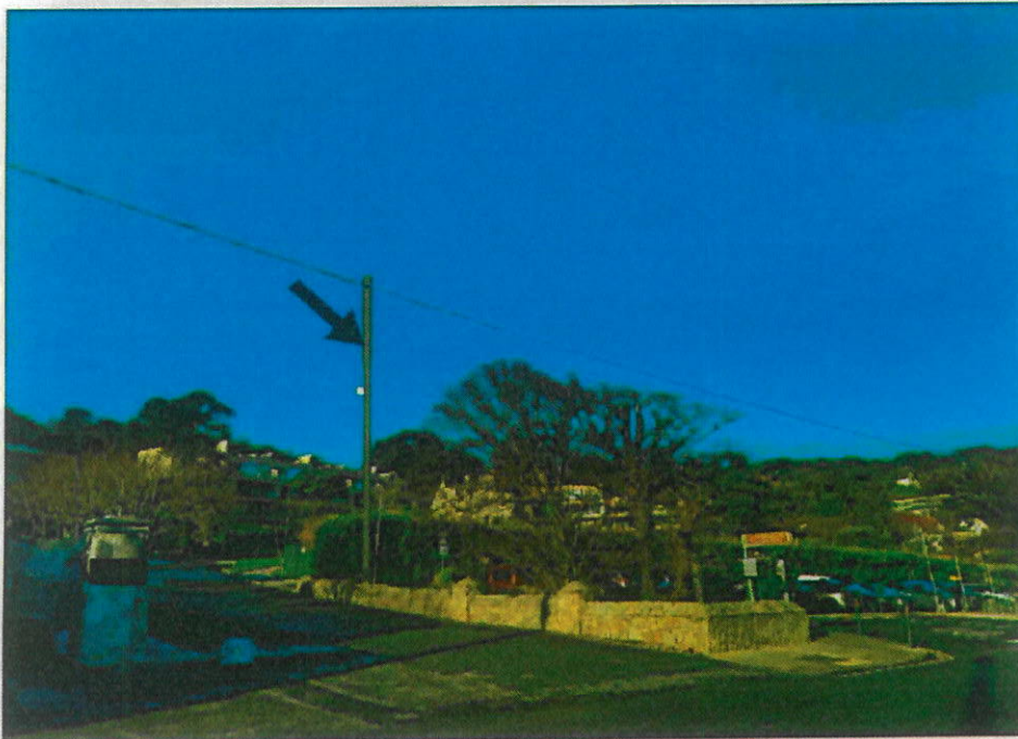
VRP6 - WITH SOLUTION IN PLACE
