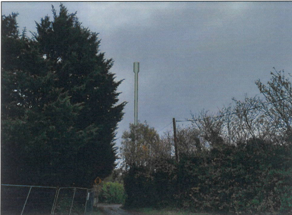
VRP3 - WITH SOLUTION IN PLACE
