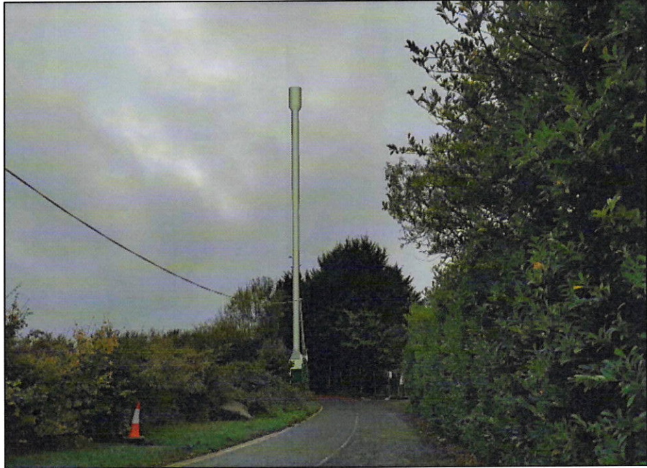
VRP4 - WITH SOLUTION IN PLACE
