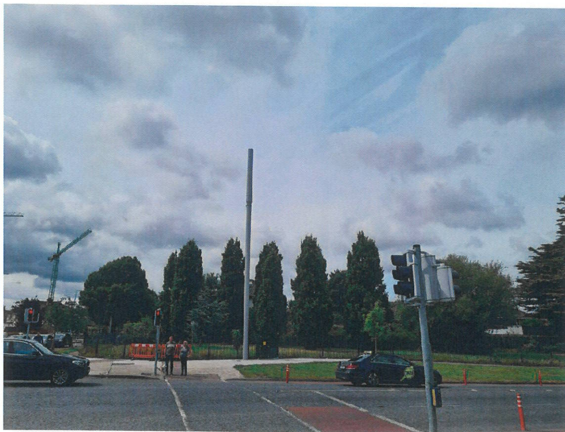
Fig 1. Existing Smart Streetpole Solution as erected in Drummartin Road, Kilmacud, D14
