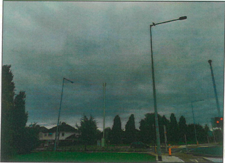
VRP9 - WITH SOLUTION IN PLACE
