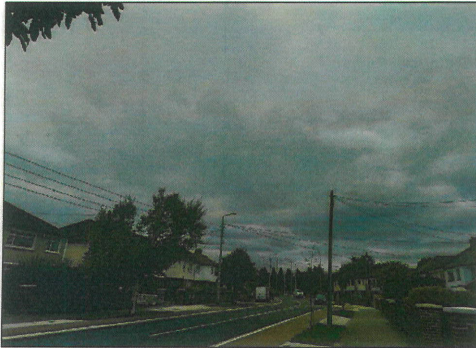
VRP11 - WITHOUT SOLUTION IN PLACE
