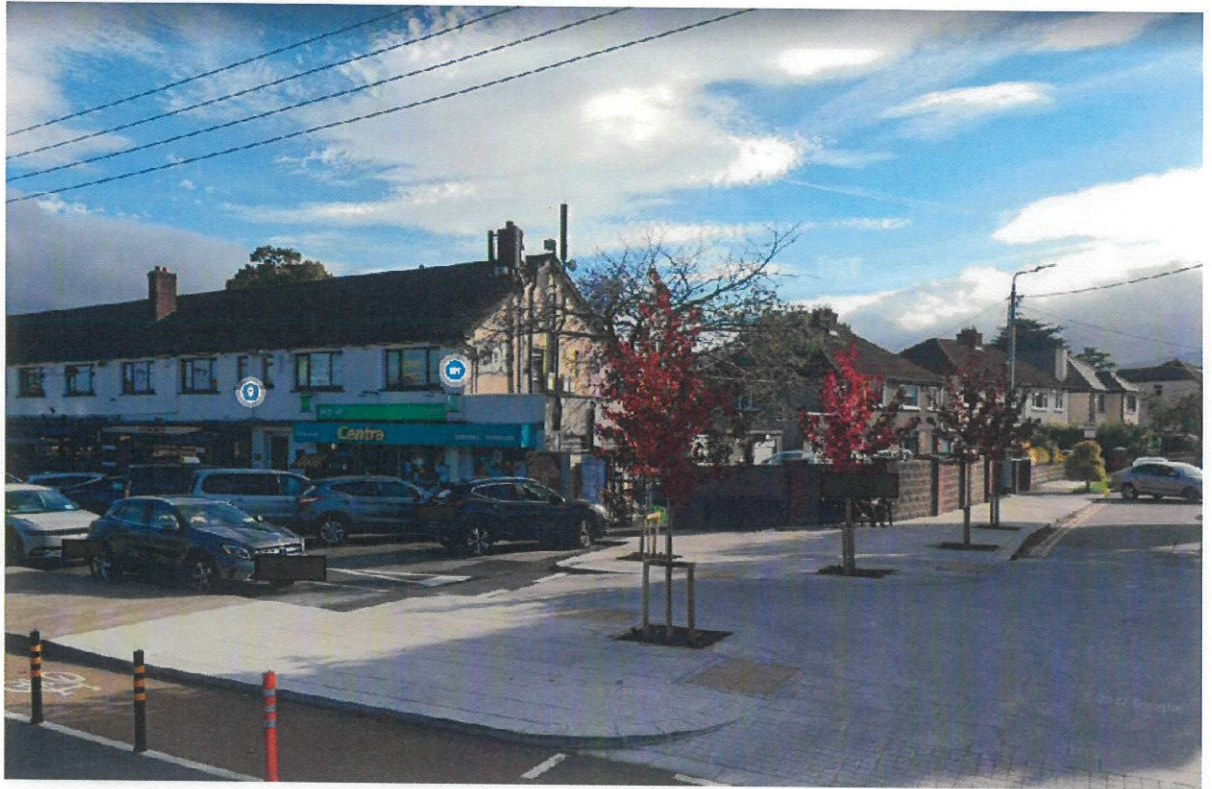
Fig 3a Existing Brady's Site DU1283 mounted to chimney/roof
