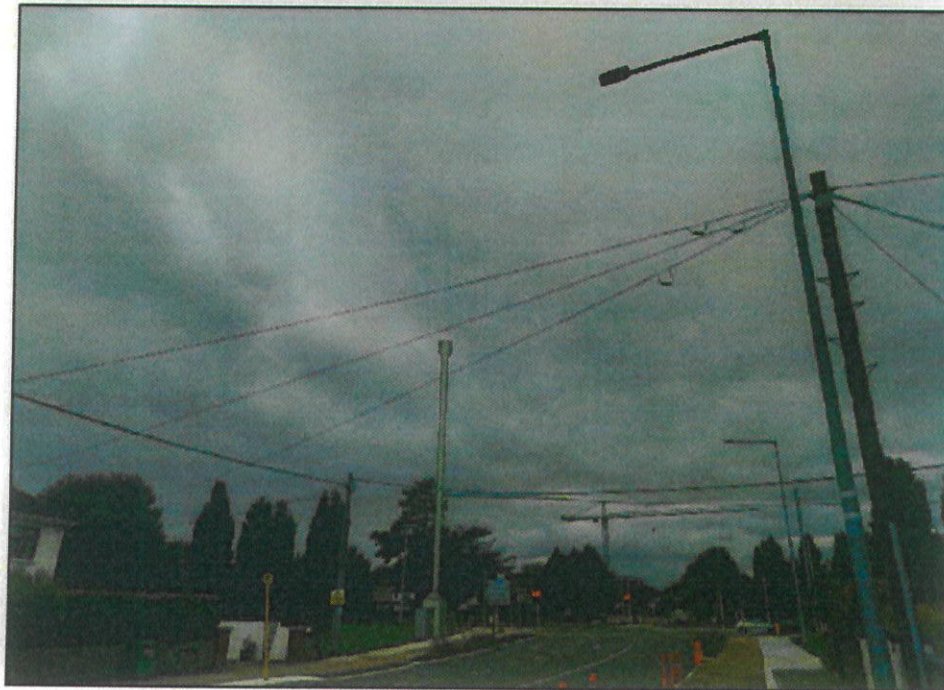
VRP10 - WITH SOLUTION IN PLACE
