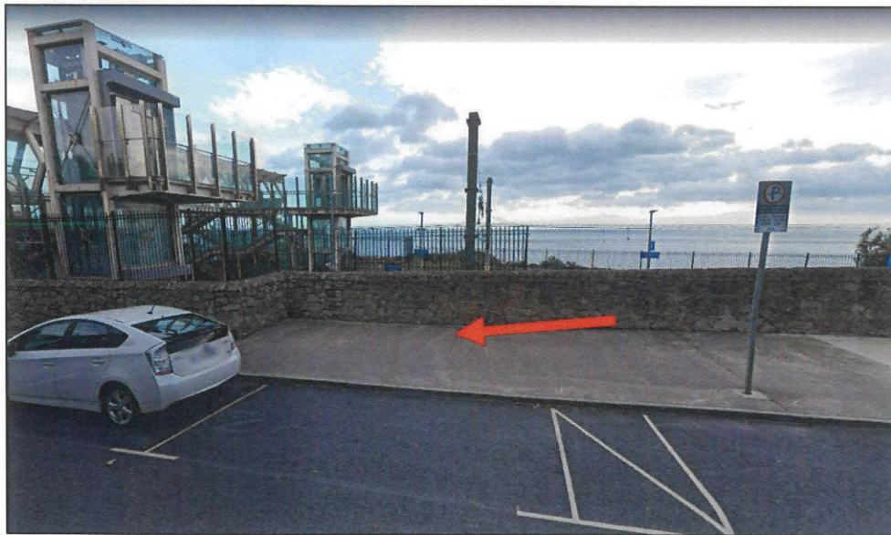
Fig No.1 Photograph of subject site.
