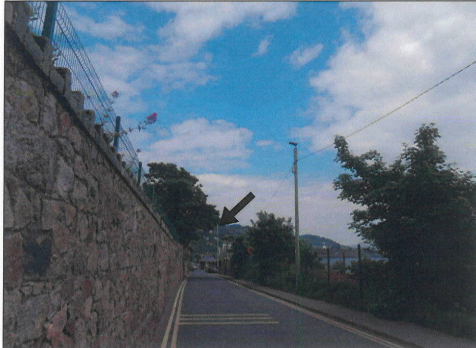
VRP1 - WITH SOLUTION IN PLACE
