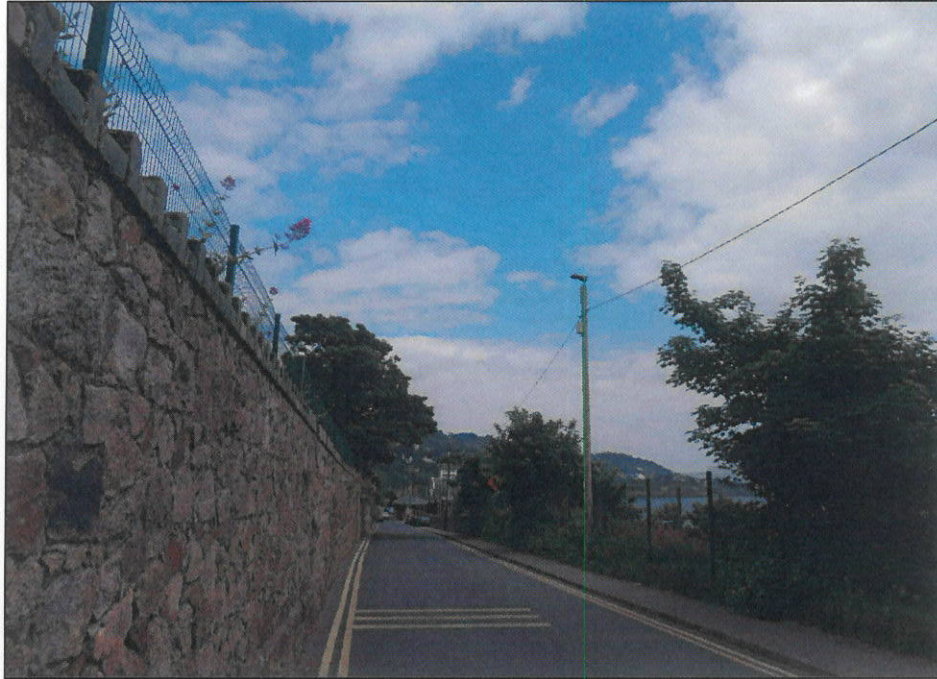
VRP1 - WITHOUT SOLUTION IN PLACE
