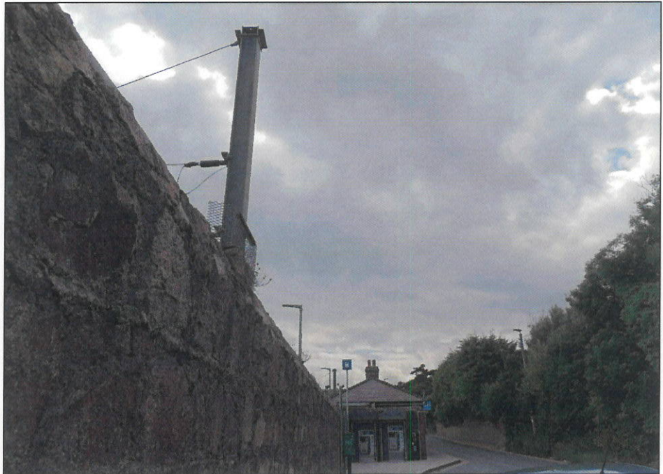
VRP4 - WITHOUT SOLUTION IN PLACE
