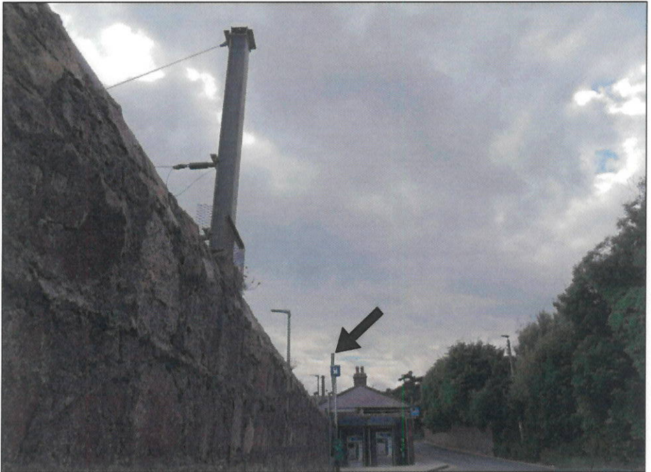
VRP4 - WITH SOLUTION IN PLACE
