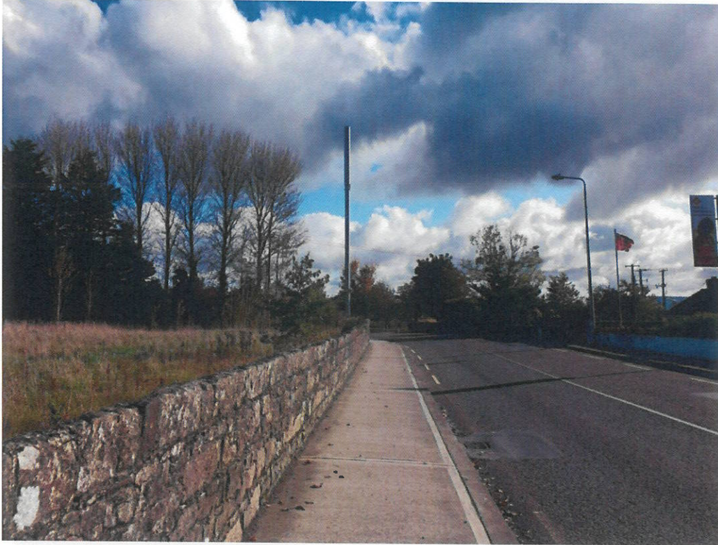
Streetworks solution at Bagenelstown, Co Carlow (Structure is Alpha 2.0 Construct)
