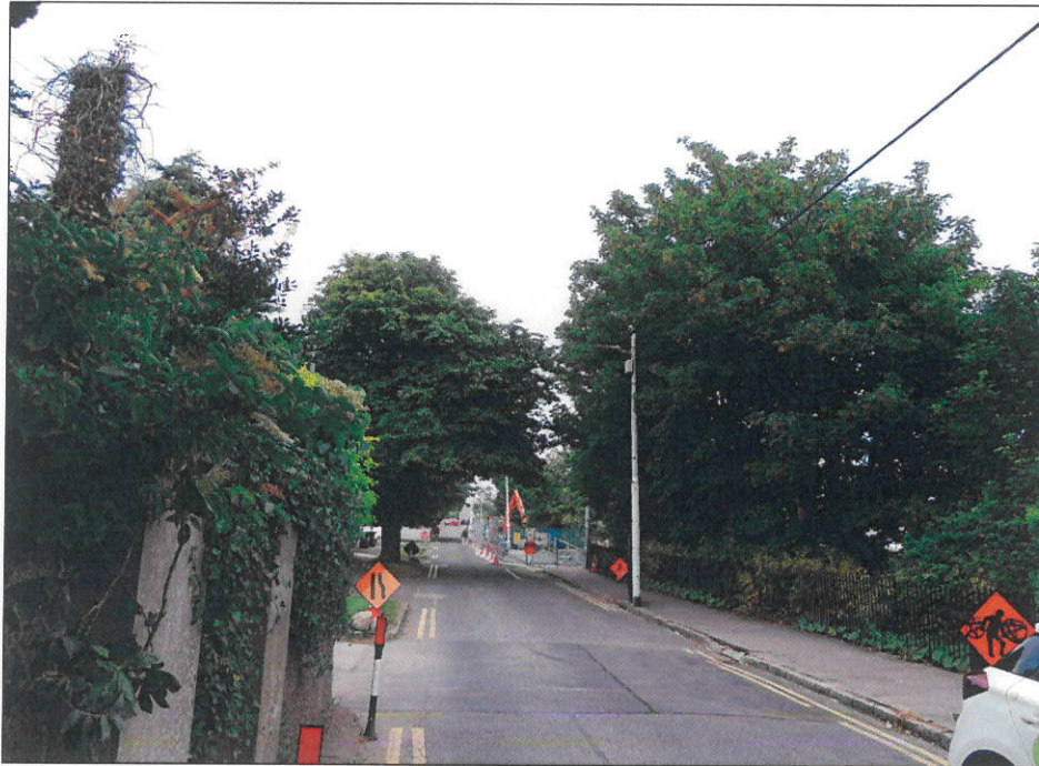
VRP5 - WITHOUT SOLUTION IN PLACE
