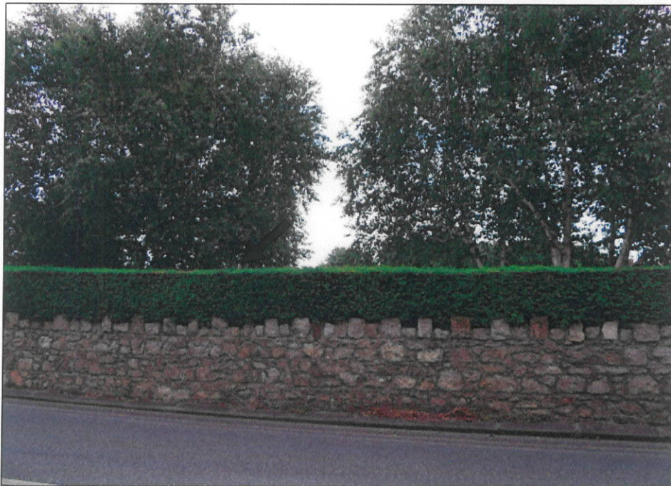
VRP1 - WITH SOLUTION IN PLACE
