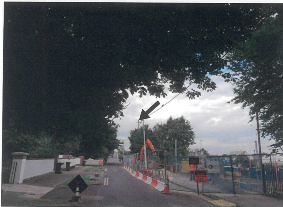
VRP6 - WITH SOLUTION IN PLACE
