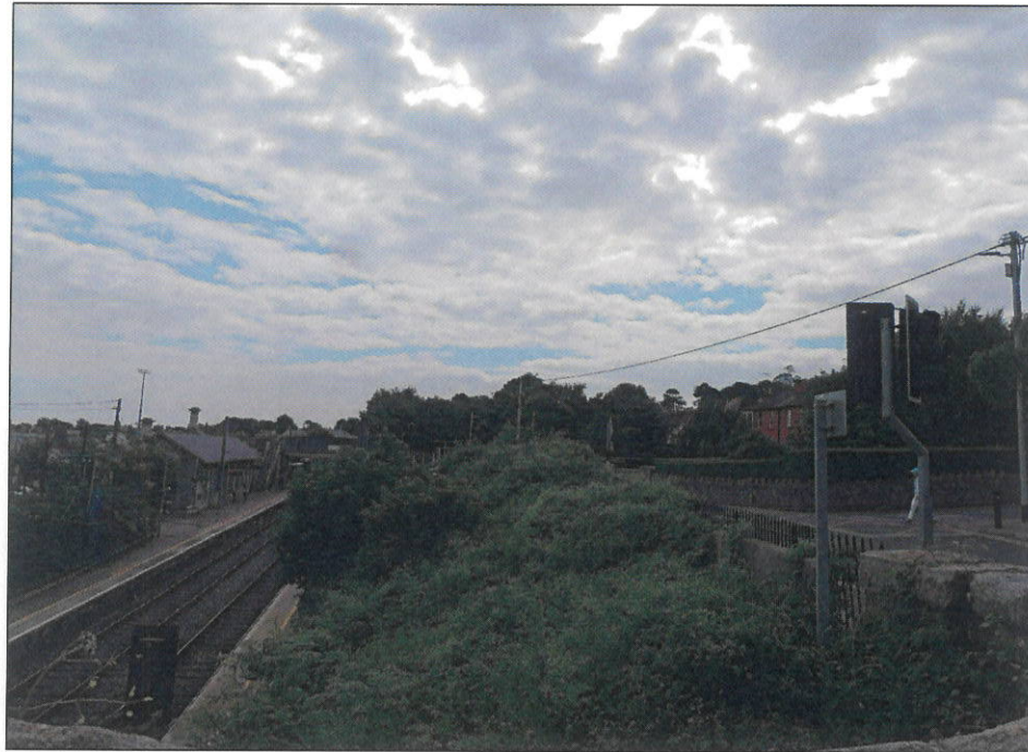
VRP3 - WITHOUT SOLUTION IN PLACE
