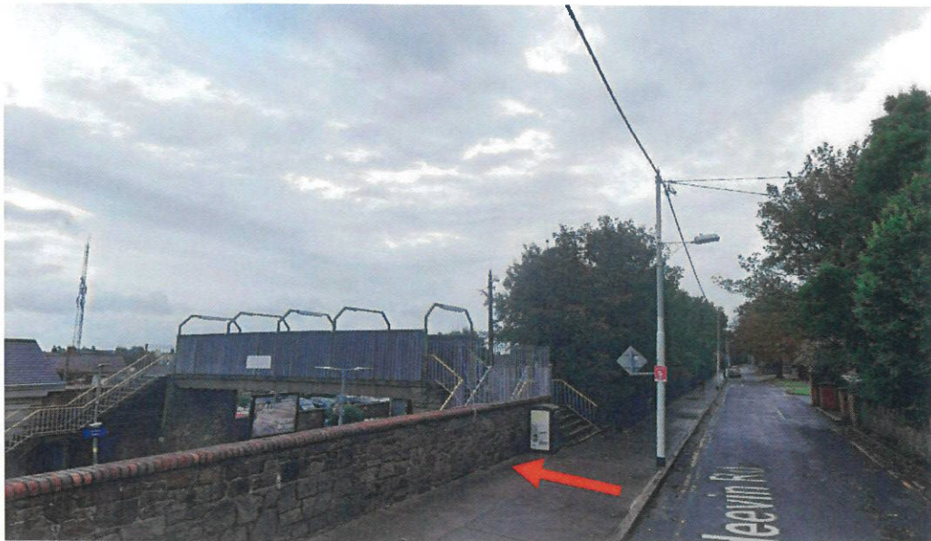
Fig No.1 Photograph of subject site (approx..) taken from the Ardeevin Rd
