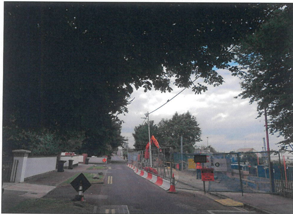
VRP6 - WITHOUT SOLUTION IN PLACE
