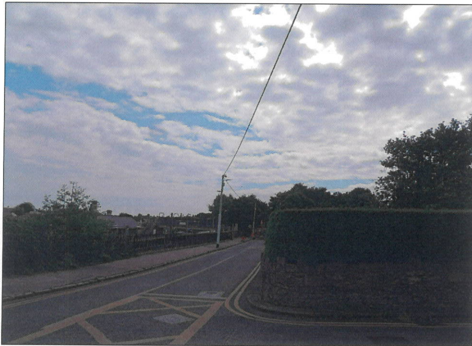
VRP2 - WITHOUT SOLUTION IN PLACE
