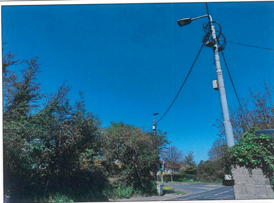
VRP3 - WITHOUT SOLUTION IN PLACE
