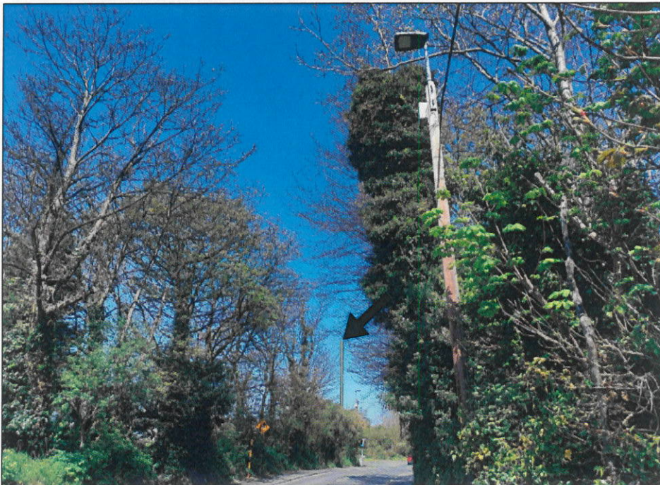
VRP2 - WITH SOLUTION IN PLACE
