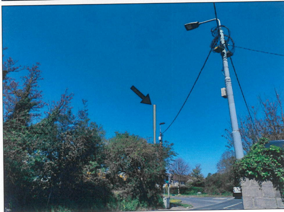
VRP3 - WITH SOLUTION IN PLACE
