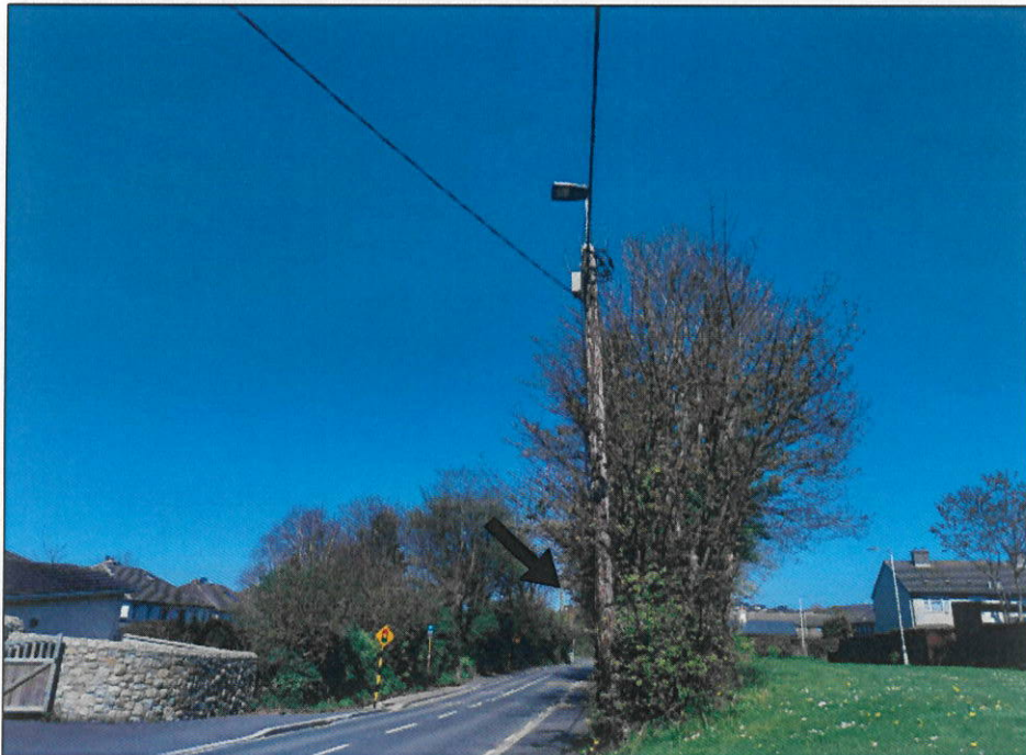
VRP1 - WITH SOLUTION IN PLACE
