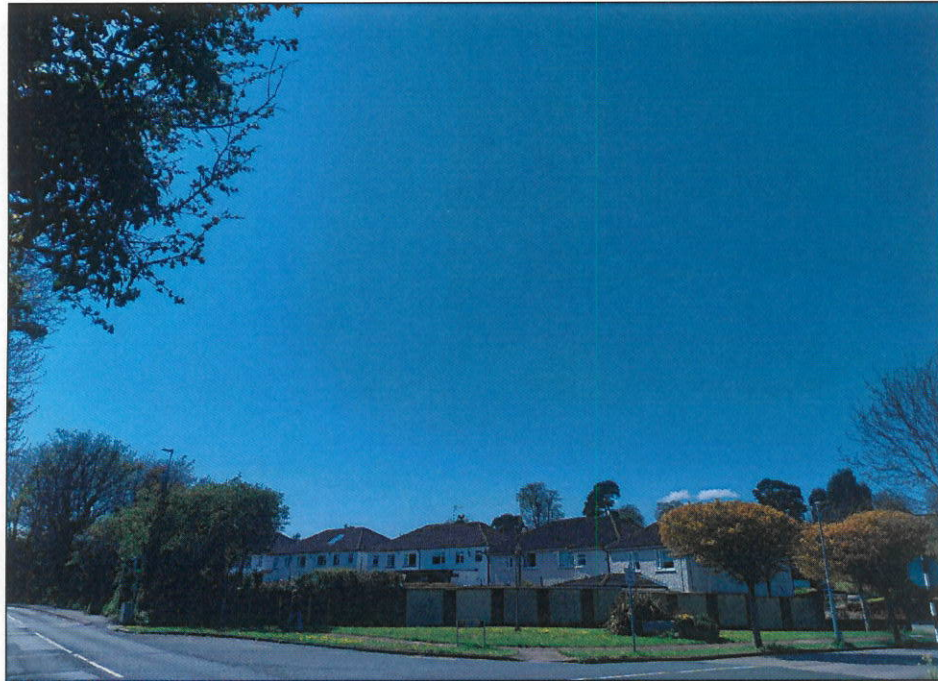
VRP6 - WITHOUT SOLUTION IN PLACE
