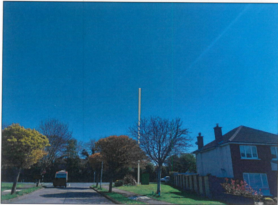
VRP8 - WITH SOLUTION IN PLACE
