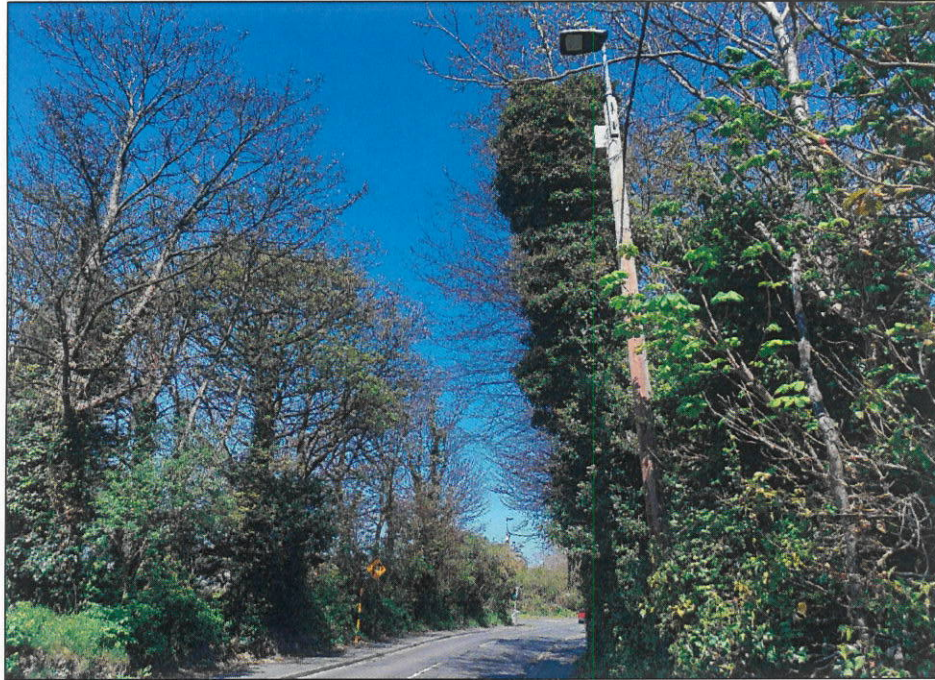
VRP2 - WITHOUT SOLUTION IN PLACE
