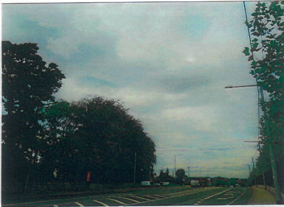
VRP3 - WITHOUT SOLUTION IN PLACE
