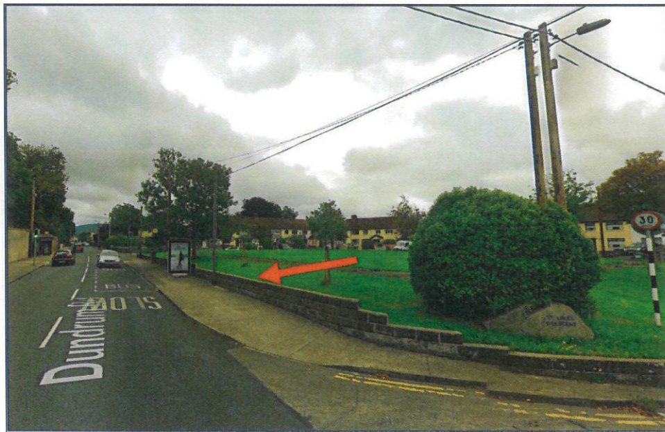
Fig No.1 Photograph of subject site taken from Dundrum Road.
