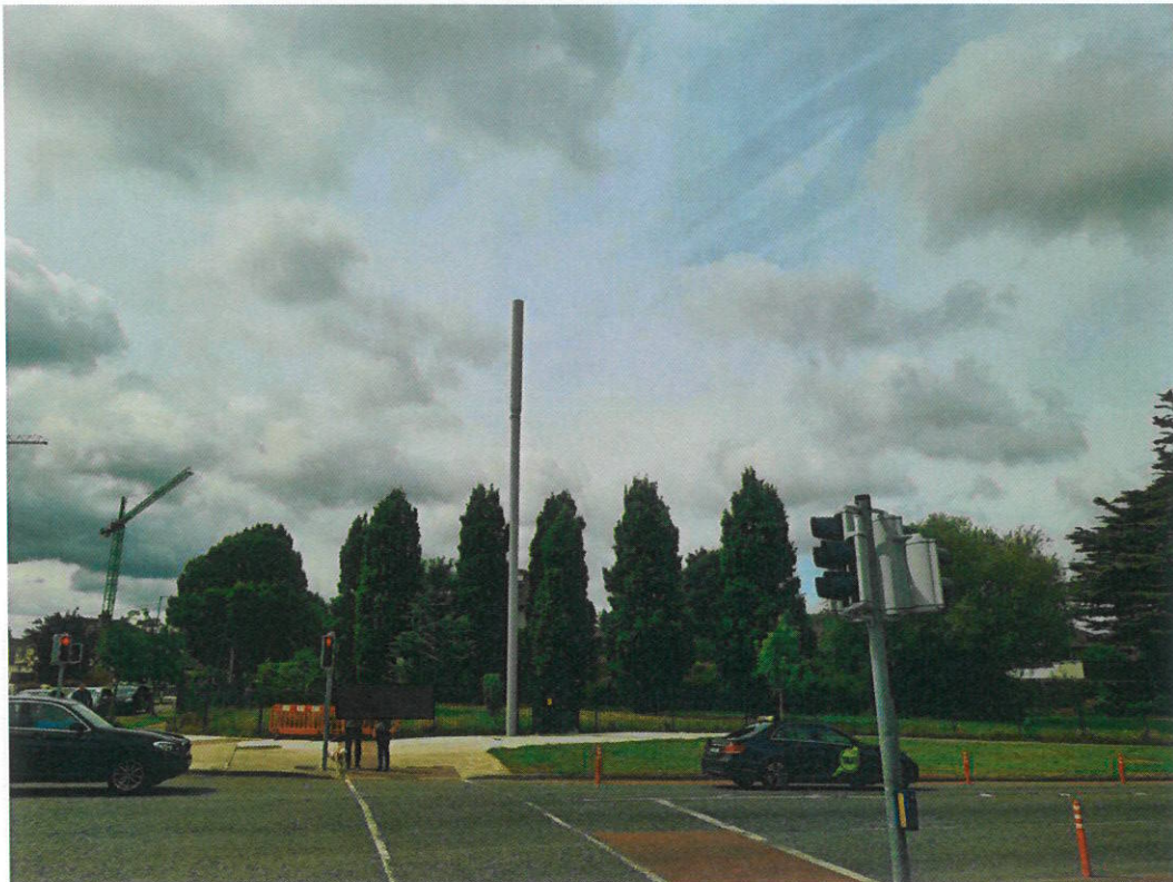
Fig 1. Existing Smart Streetpole Solution as erected in Drummartin Road, Kilmacud, D14
