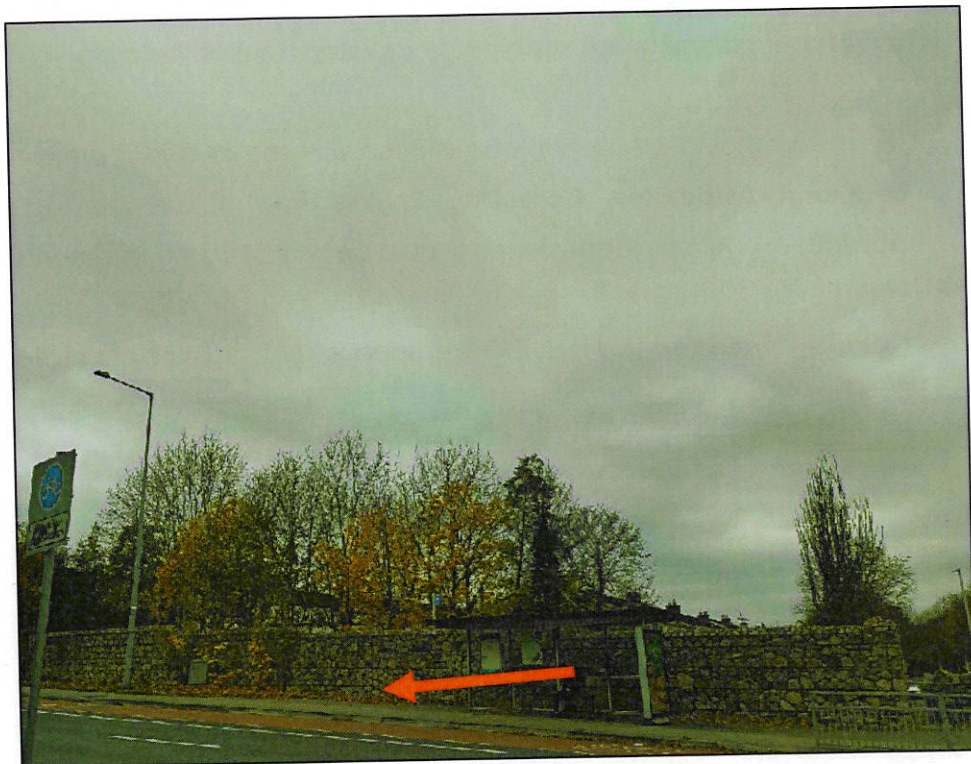
Fig No.1 Photograph of subject site taken from Kilmacud Road Upper.
