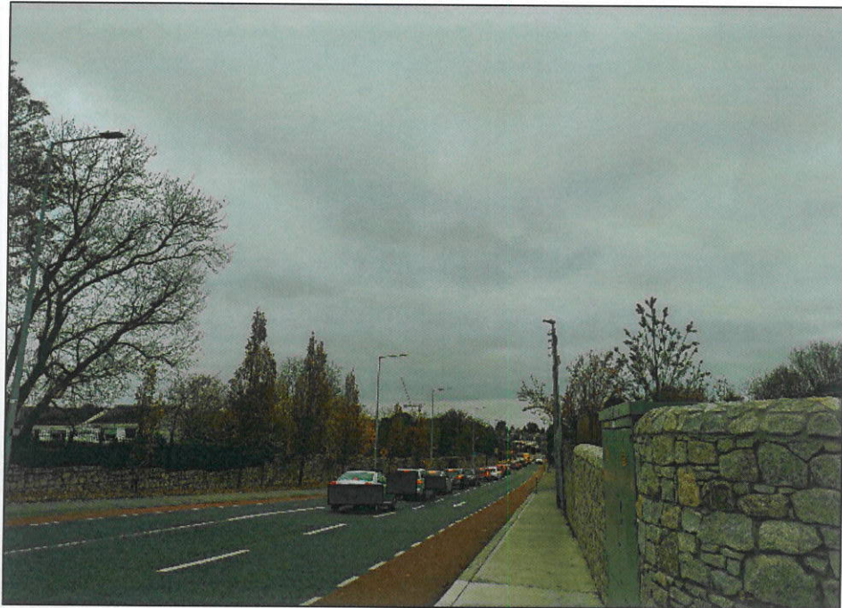
VRP2 - WITHOUT SOLUTION IN PLACE
