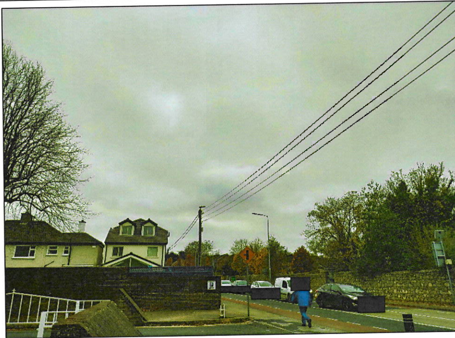
VRP1 - WITHOUT SOLUTION IN PLACE
