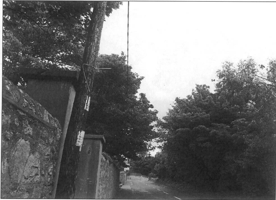
VRP1 - WITHOUT SOLUTION IN PLACE
