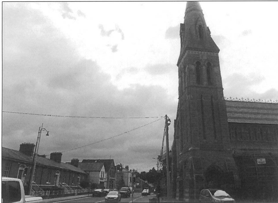
VRP1 - WITHOUT SOLUTION IN PLACE
