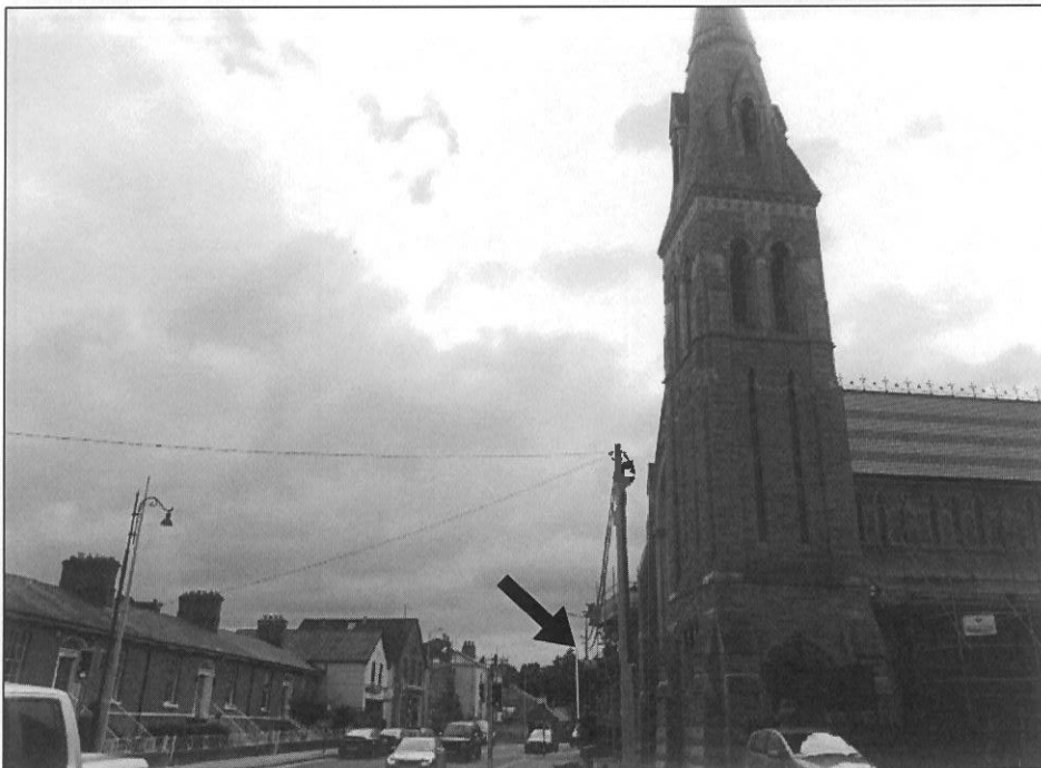
VRP1 - WITH SOLUTION IN PLACE
