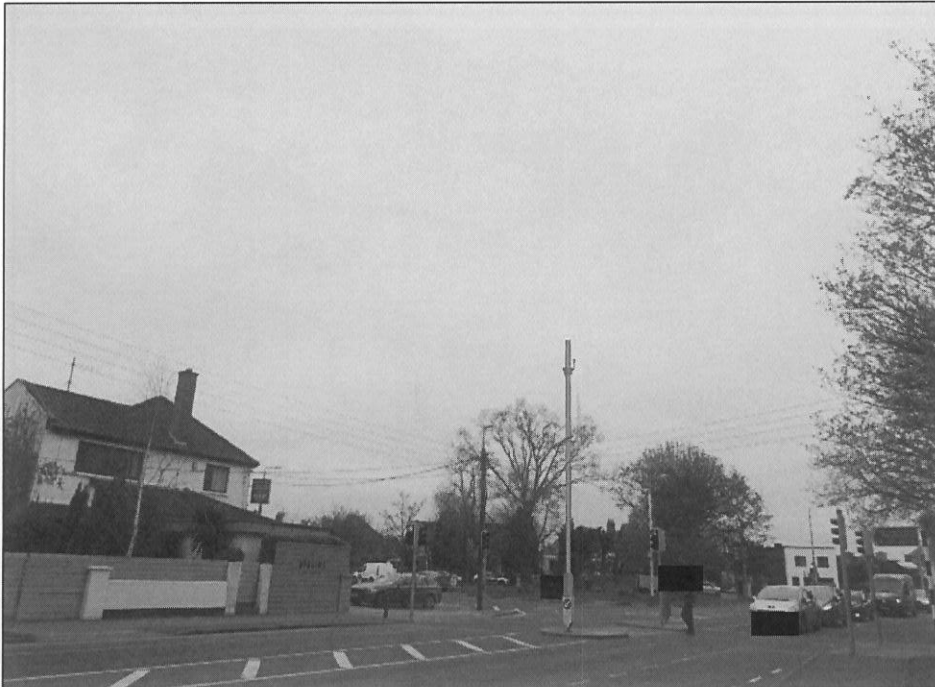
VRP3 - WITH SOLUTION IN PLACE
