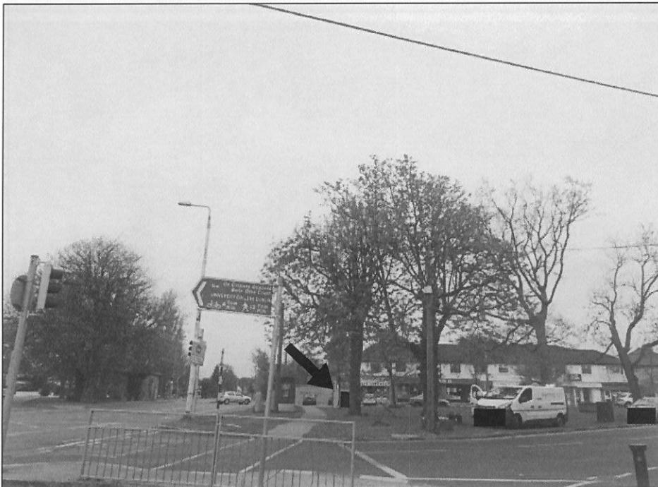
VRP9 - WITH SOLUTION IN PLACE
