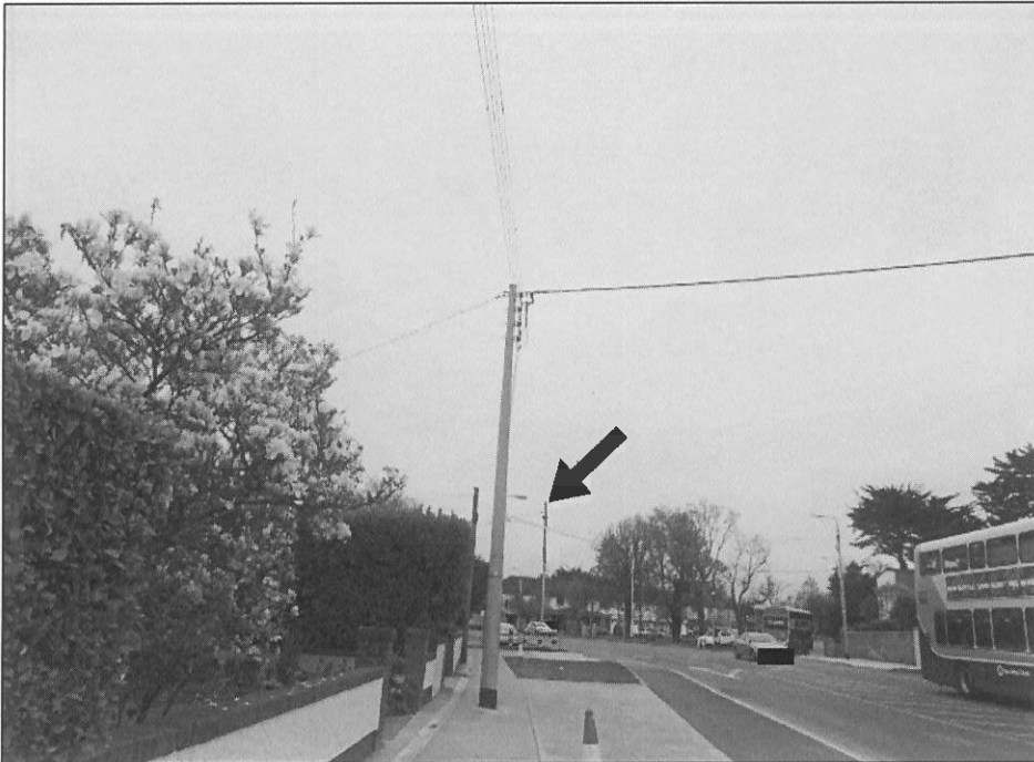
VRP5 - WITH SOLUTION IN PLACE
