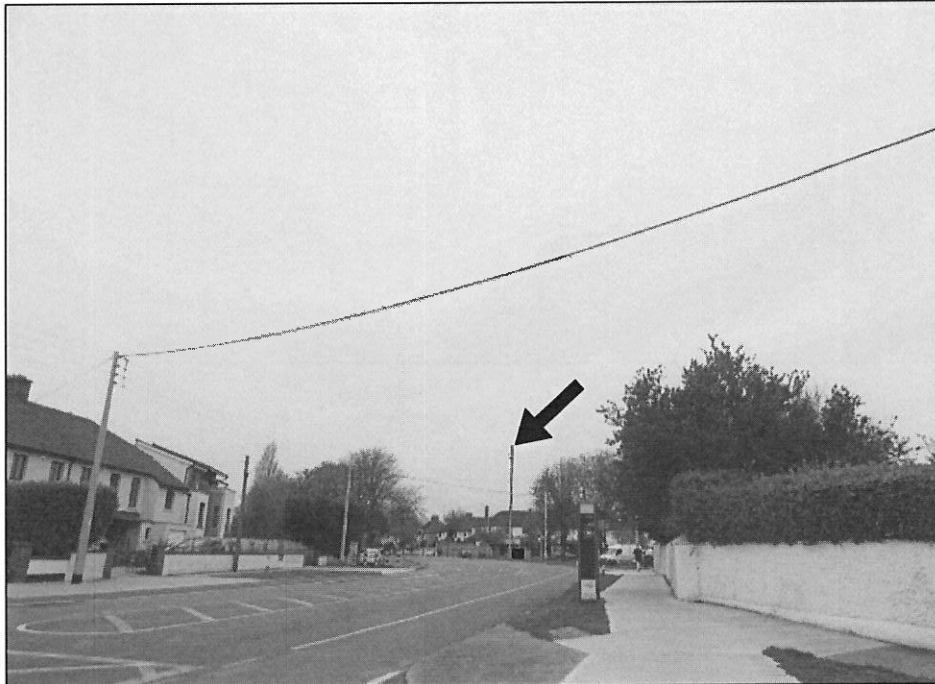
VRP8 - WITH SOLUTION IN PLACE
