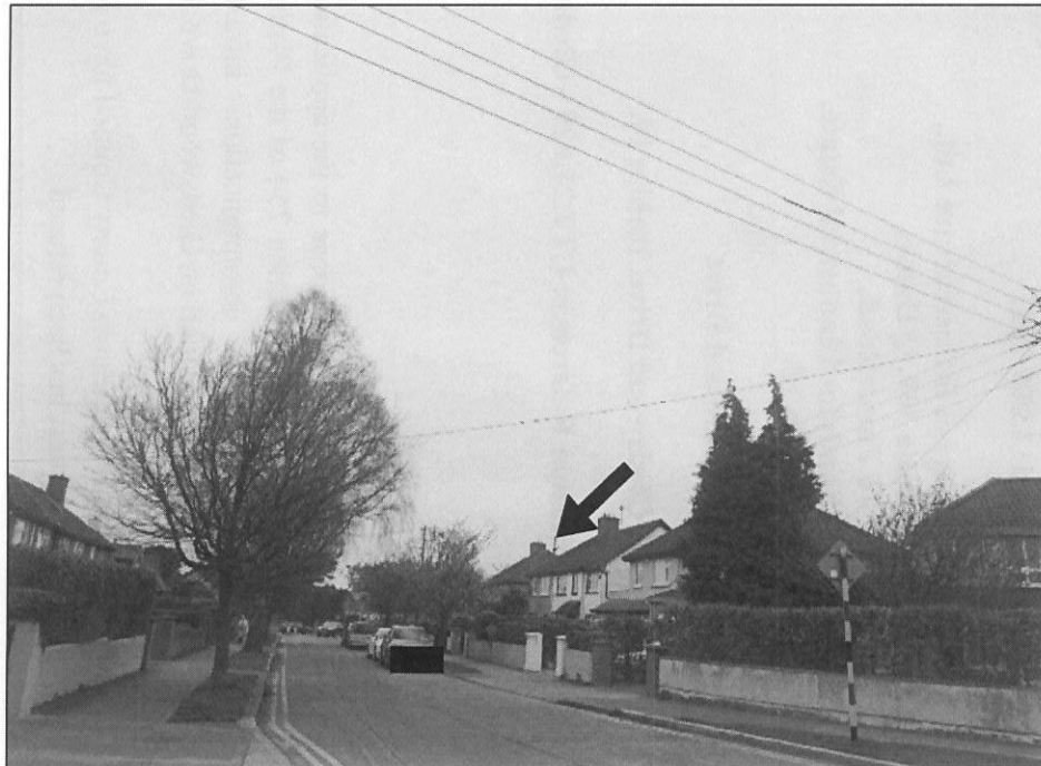
VRP13 - WITH SOLUTION IN PLACE
