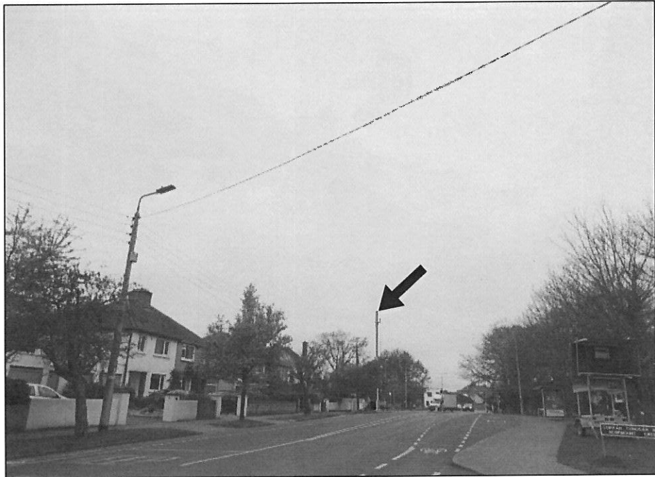
VRP2 - WITH SOLUTION IN PLACE
