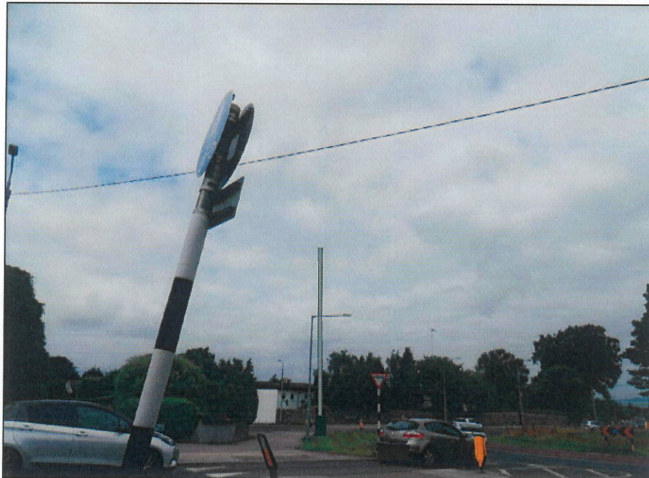
VRP3 - WITH SOLUTION IN PLACE
