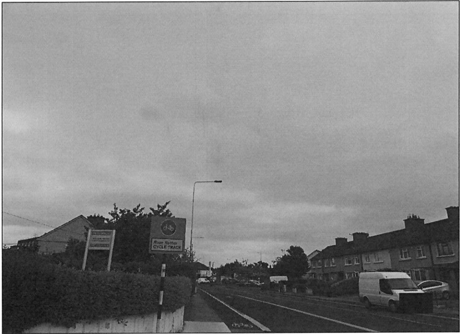
VRP2 - WITHOUT SOLUTION IN PLACE
