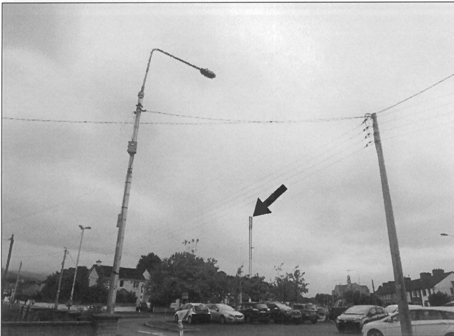
VRP5 - WITH SOLUTION IN PLACE
