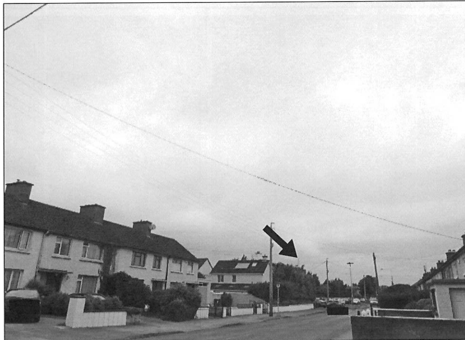
VRP6 - WITH SOLUTION IN PLACE
