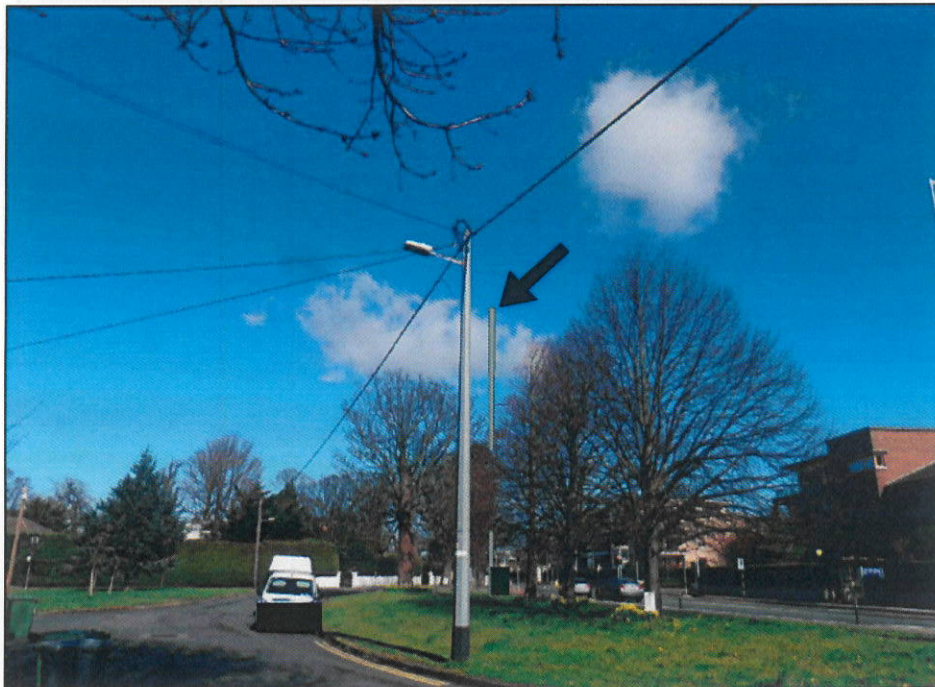
VRP4 - WITH SOLUTION IN PLACE
