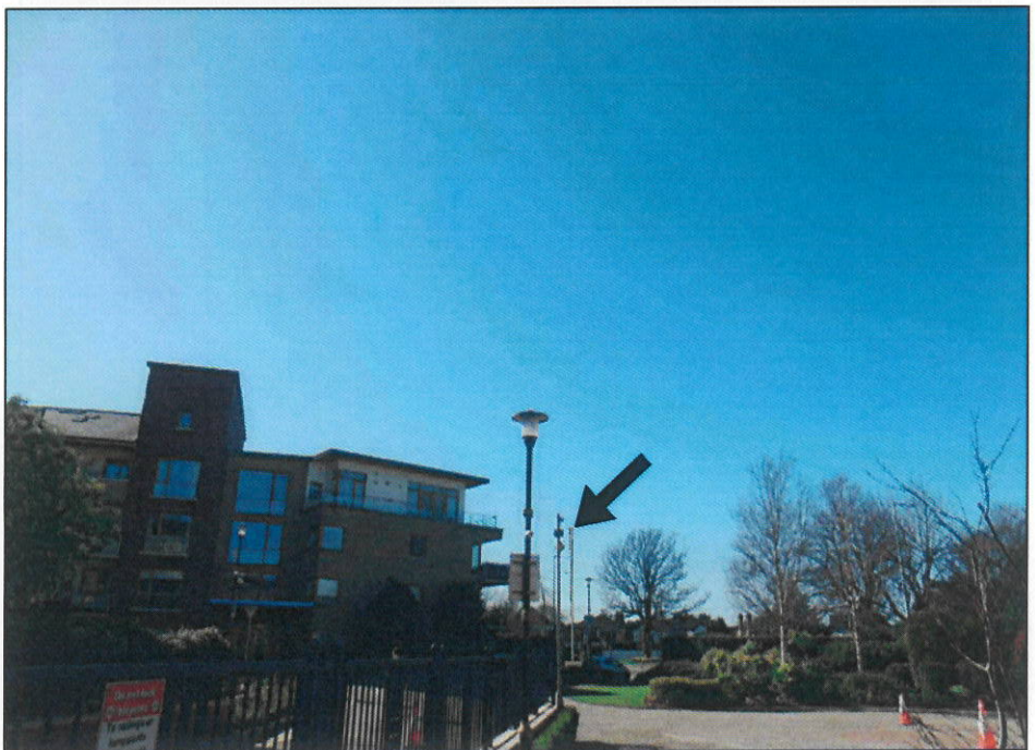
VRP16 - WITH SOLUTION IN PLACE
