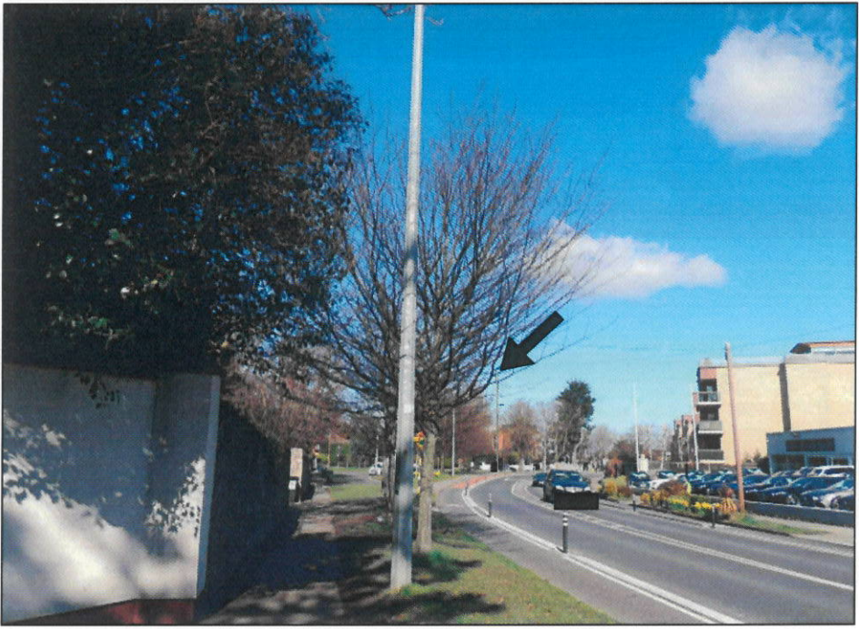
VRP2 - WITH SOLUTION IN PLACE
