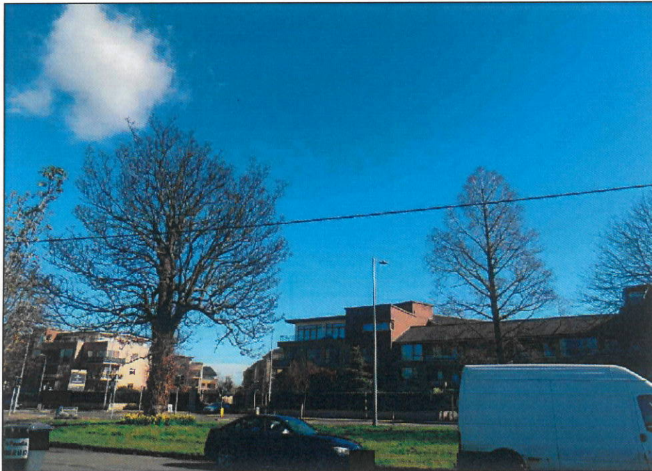
VRP5 - WITHOUT SOLUTION IN PLACE
