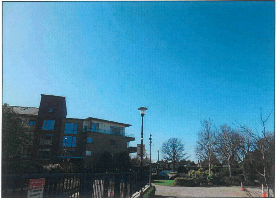
VRP16 - WITHOUT SOLUTION IN PLACE
