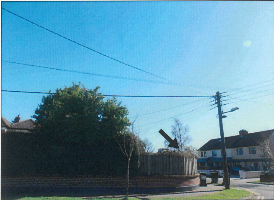
VRP11 - WITH SOLUTION IN PLACE
