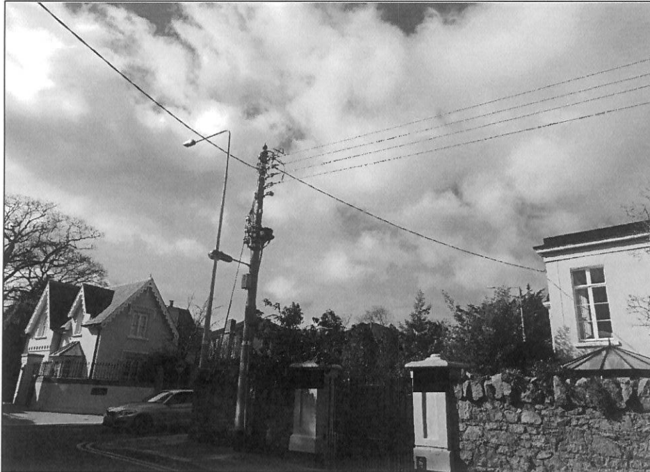
VRP3 - WITHOUT SOLUTION IN PLACE
