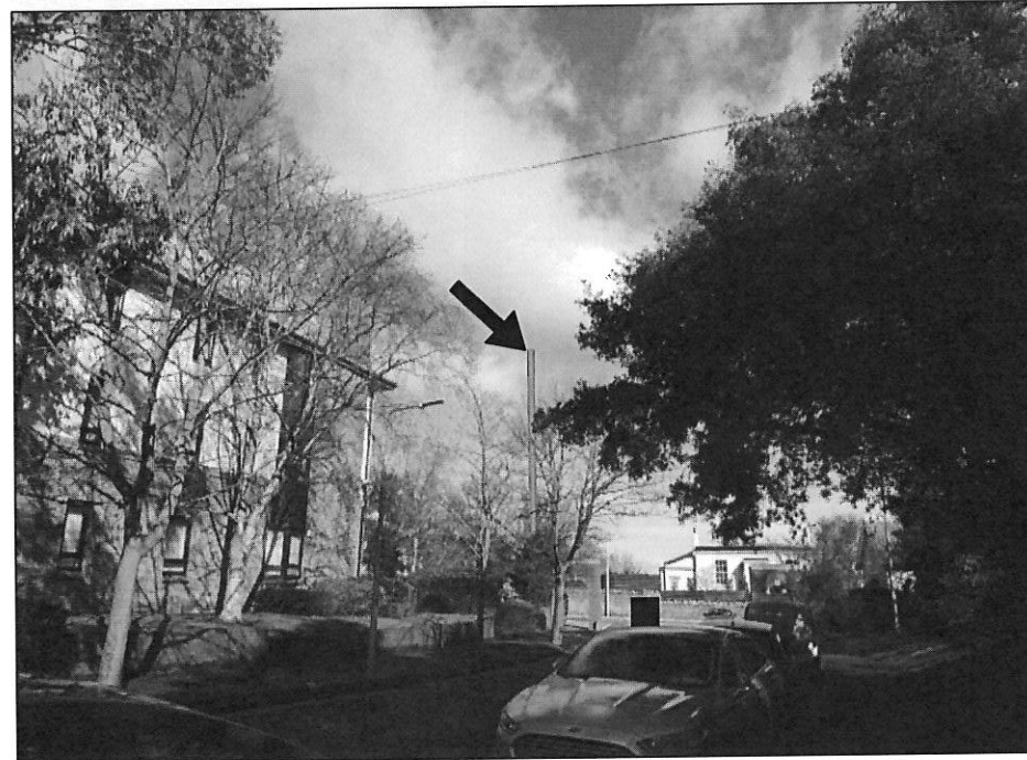
VRP10 - WITH SOLUTION IN PLACE
