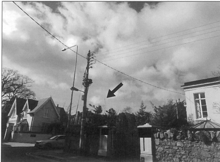
VRP3 - WITH SOLUTION IN PLACE
