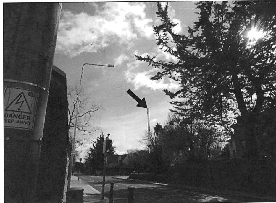
VRP6 - WITH SOLUTION IN PLACE
