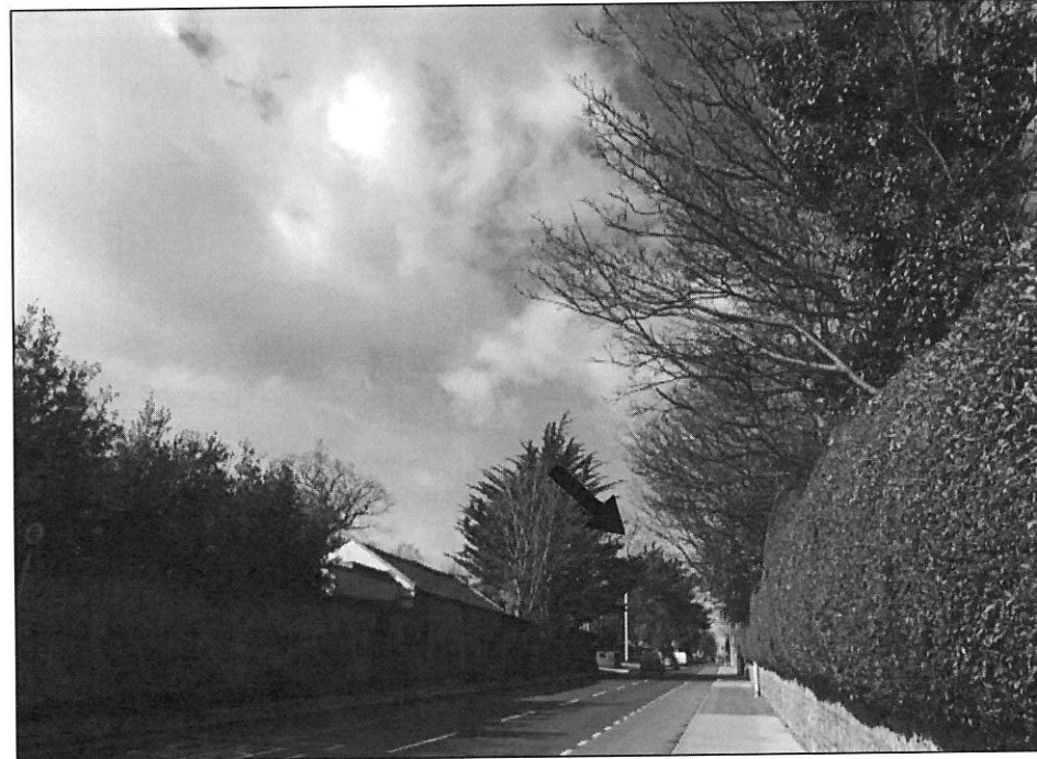
VRP2 - WITH SOLUTION IN PLACE
