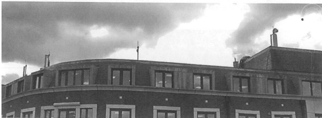
Image 5 Existing eir Mobile rooftop site (co-located ) in Stillorgan ComReg Site ID: 1312
