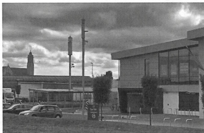
Image 6 Closest eir Mobile installation on Three's structure ComReg Site ID1218 Registry Ref: D17A/0499
