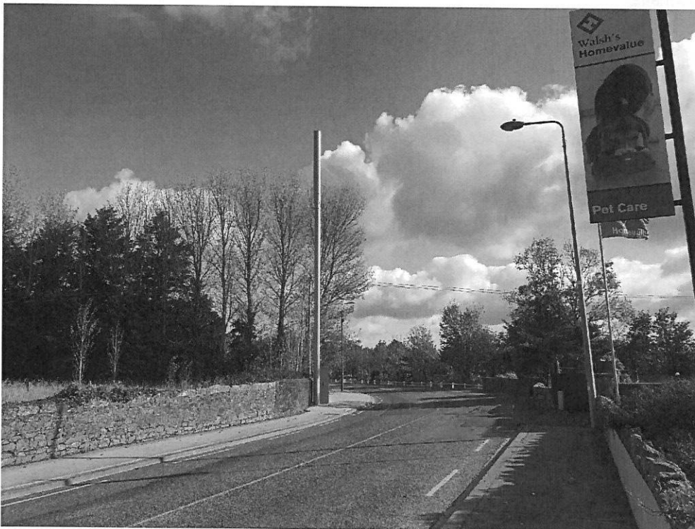
Fig 1. Existing Smart Streetpole Solution as erected in Bagenalstown, Co Carlow
