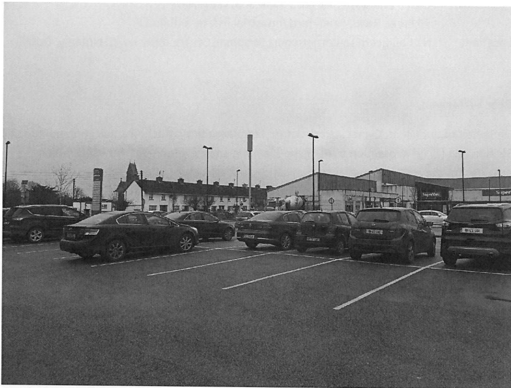
Fig 1. Existing Smart Streetpole Solution as erected in Mountmellick, Co Laois
