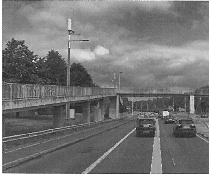
Image 5: Existing street solutions on Cabinteely By Pass from Google Earth
