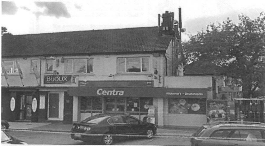
Image 1 Existing eir Mobile and Three rooftop installation on Drummartin Road
