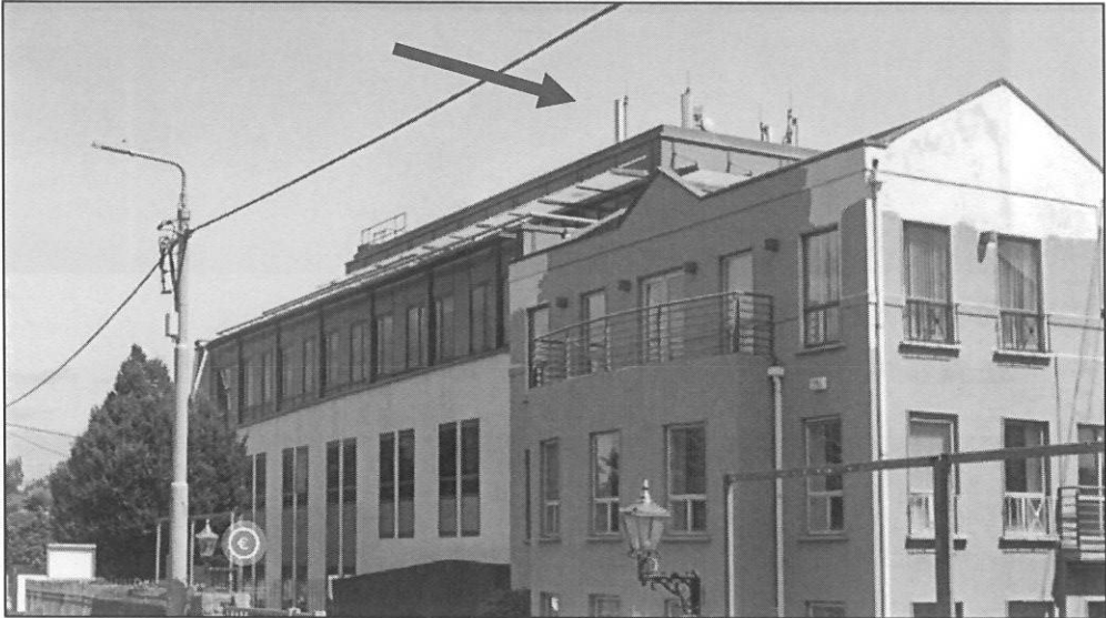
Fig No.8 Located on roof of Carysfort House.
