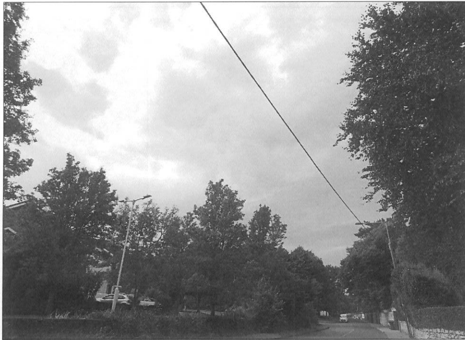
VRP2 - WITHOUT SOLUTION IN PLACE
