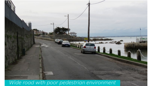
Wide road with poor pedestrian environment
