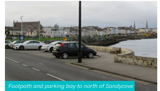
Footpath and parking bay north of Sandycove
