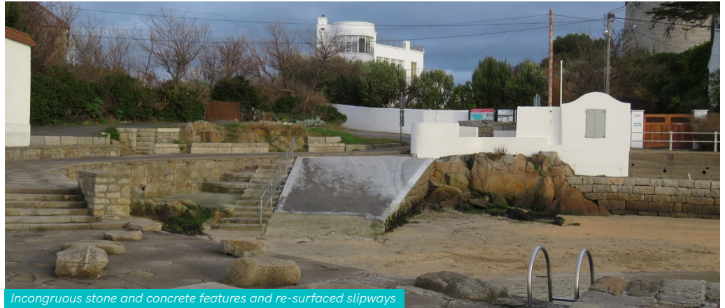
Incongruous stone and concrete features and re-surfaced slipways
