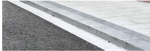
Asphalt with granite chipping, granite setts channel and kerb for other roadway in vicinity of the Harbours
