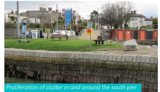
Proliferation of clutter in and around the south pier
