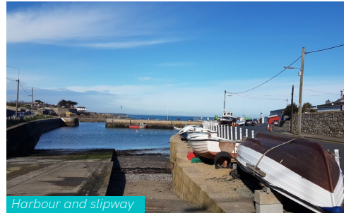
Harbour and slipway
