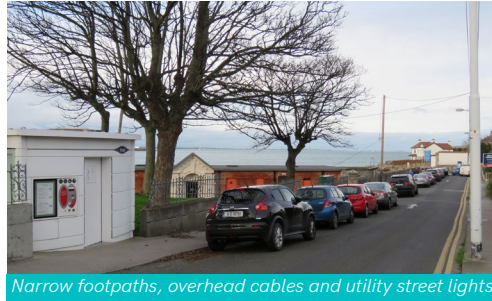
Narrow footpaths, overhead cables and utility street lights
