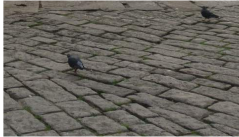
Granite setts for around the piers and along Sandycove Point (as far as the Geragh Haus)
