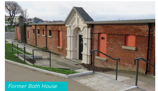
Former Bath House
